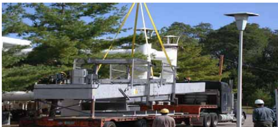
BAR SCREENS BEING OFF-LOADED
