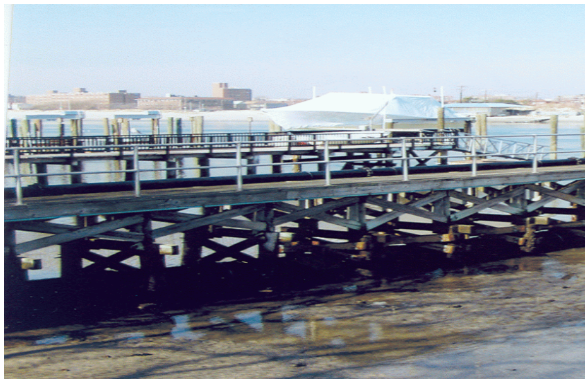
NEW SUPPORT TIMBERS AND HARDWARE FOR OUTFALL PIER
