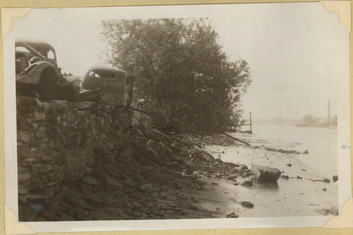
Undermined Retaining Wall North Arlington Junk Yard River Road, North Arlington, New Jersey August 29, 1948
