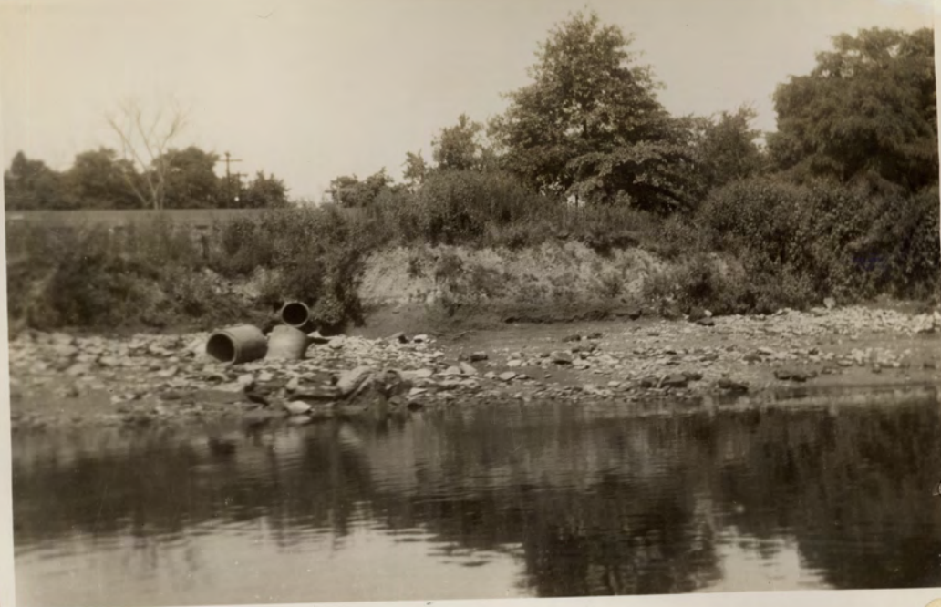
Storm Sewer Outlet Washing Away At Passaic City Dock Passaic, New Jersey August 29, 1948
