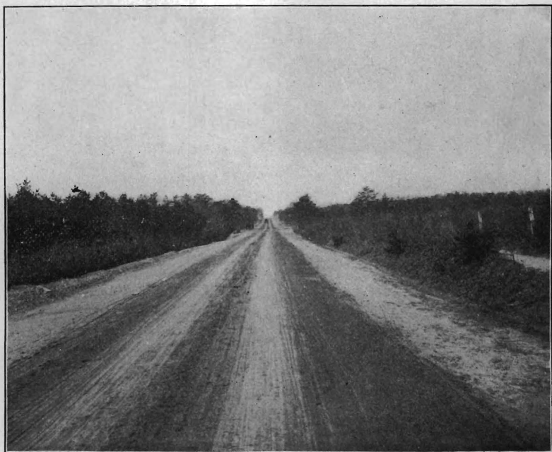
Corliss Avenue, Monmouth Co., after improvement.
