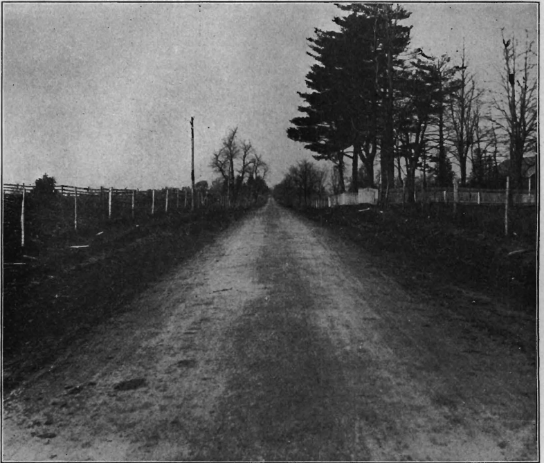
Manalapan and Freehold road, Monmouth Co., after improvement.
