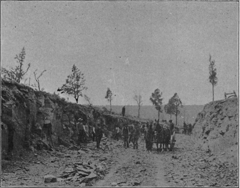
Marshall's Corner and Woodsville road, Mercer Co., working on 15-foot rock cut, during construction.
