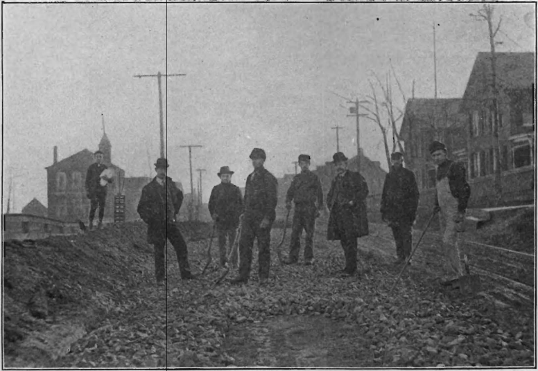
Sayreville road, Middlesex Co., laying first course.
