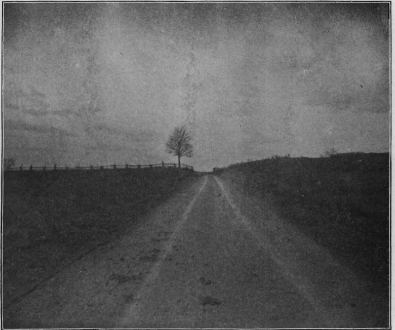
Stewartsville road, Warren Co., after improvement.
