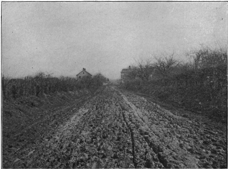
Neshanic road, Somerset Co., before improvement.
