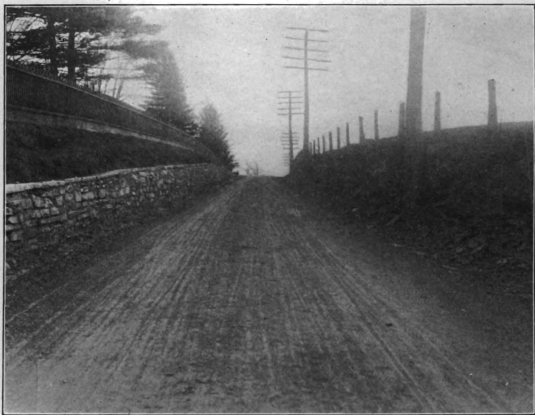
New Brunswick and Bound Brook road, Middlesex Co., after improvement.
