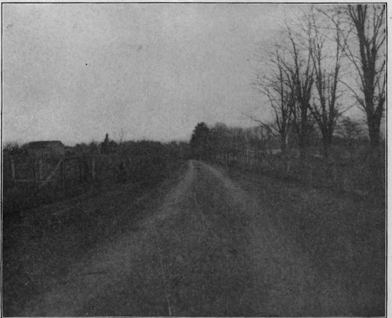
Looking toward Crosswicks on Bordentown and Crosswicks turnpike, Burlington Co., after completion.
