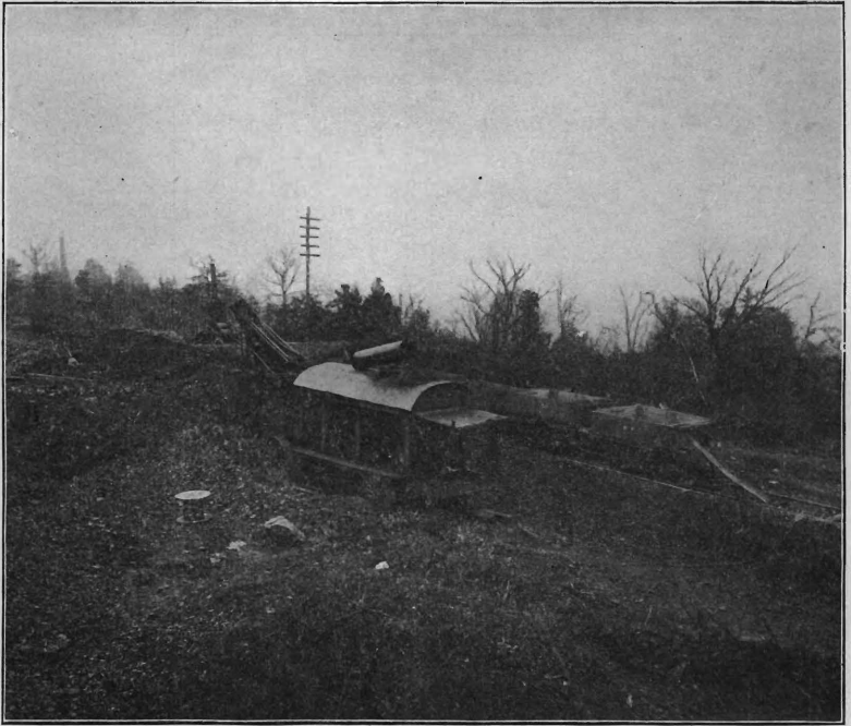
Excavation on Belleville turnpike, Bergen Co. This is where we are getting our filling. Showing the steam shovel and engine for hoisting the cars from the bottom of the hill.
