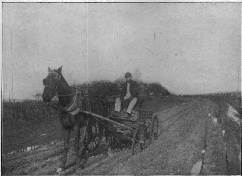
Neshanic road, Somerset Co., before improvement.
