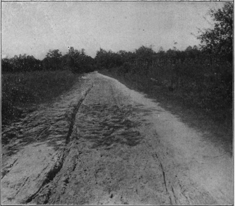
New Gretna road, Burlington Co., before improvement.
