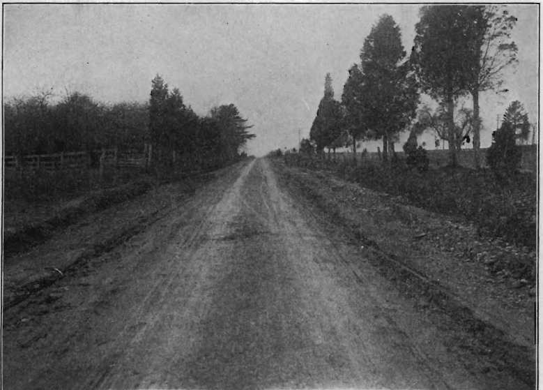
Columbus and Burlington road, Burlington Co., after improvement.
