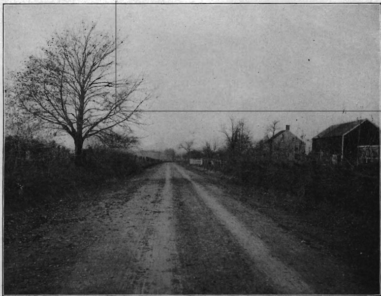
Neshanic road, Somerset Co., after improvement.
