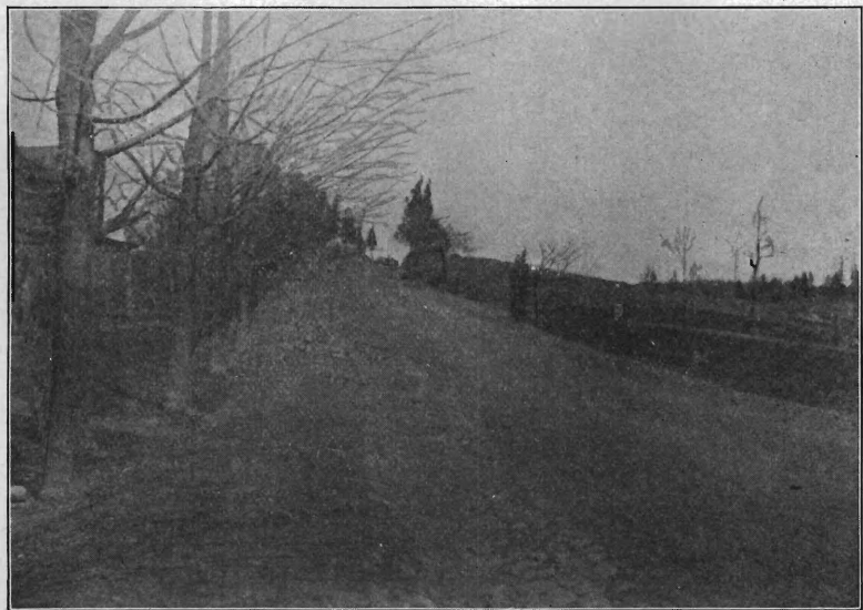
Squaw Brook road, Passaic Co., after improvement.
