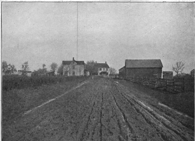
Neshanic road, Somerset Co., before improvement.
