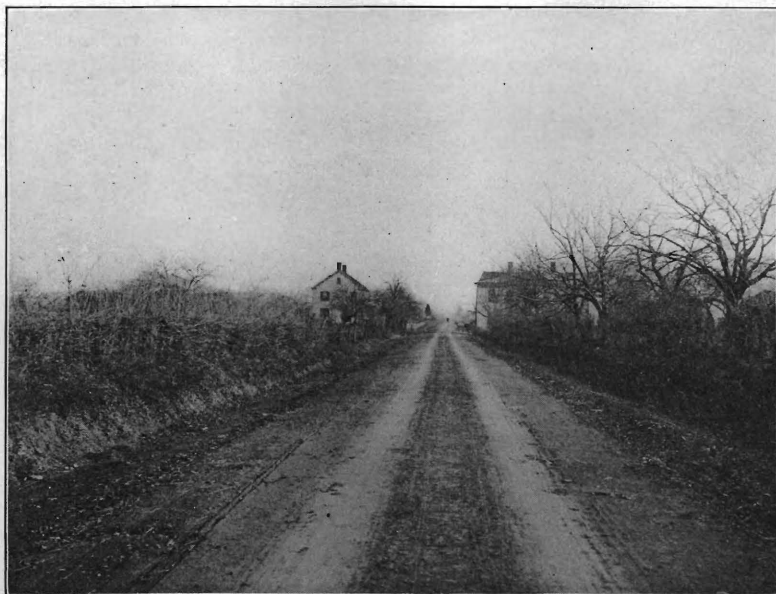
Neshanic road, Somerset Co., after improvement.
