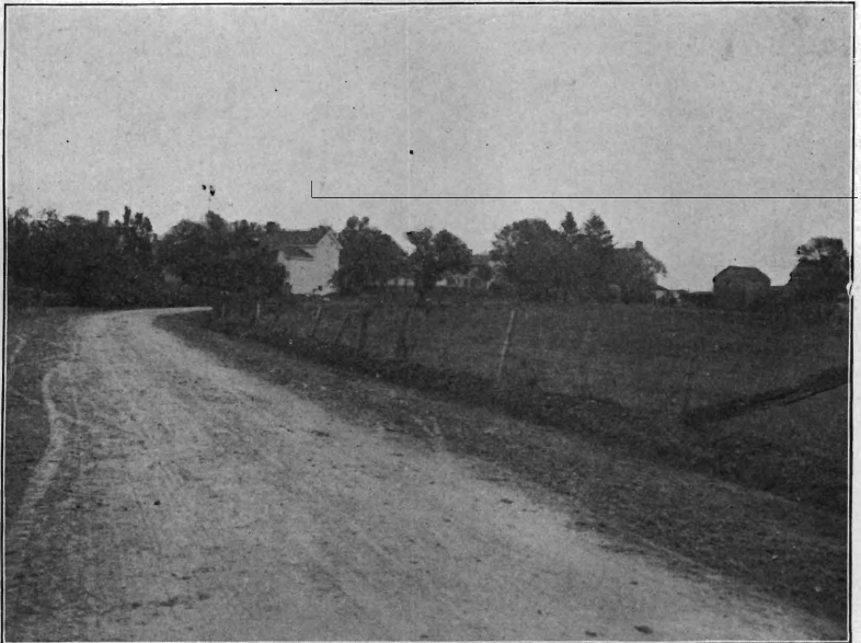
Marshall's Corner and Woodsville road, Mercer Co., after completion.
