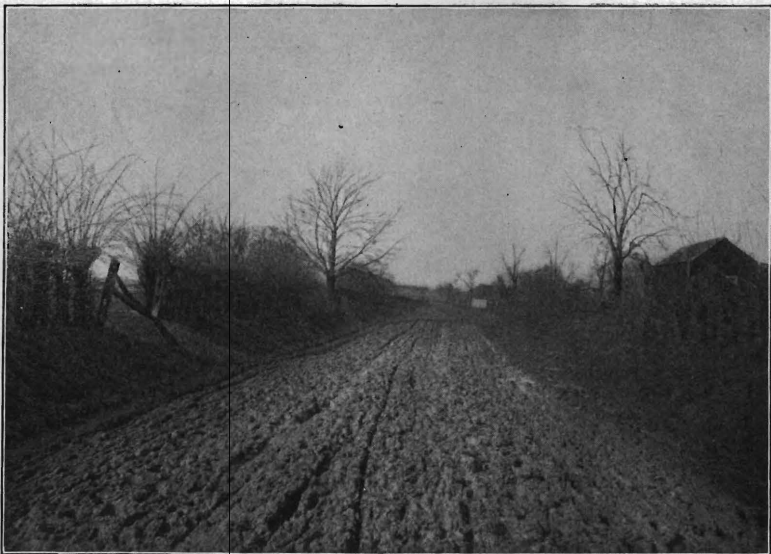
Neshanic road, Somerset Co., before improvement.
