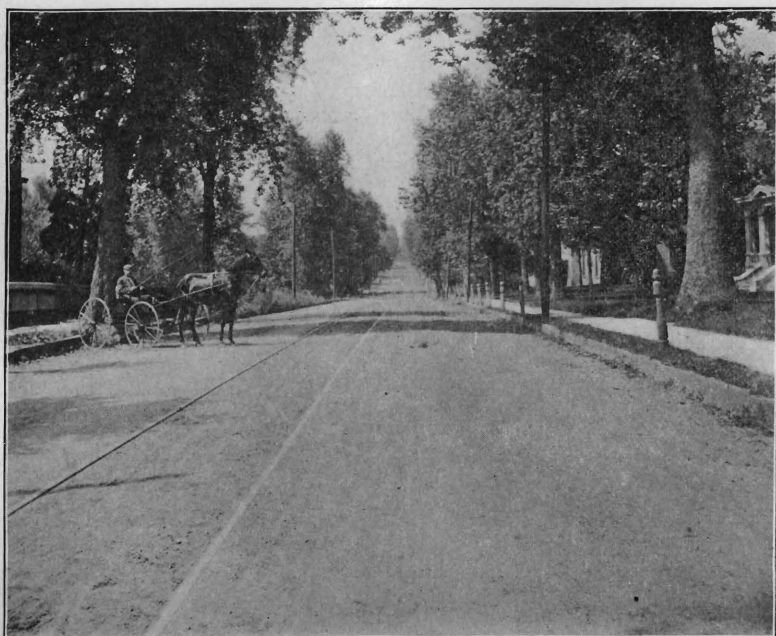
Main Street, Matawan, Monmouth Co., after improvement.
