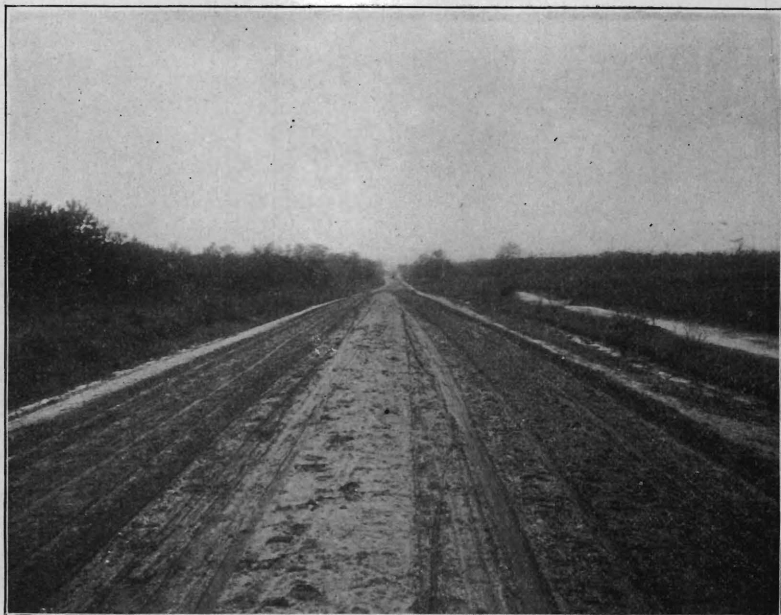
Corliss Avenue, Monmouth Co., before improvement.
