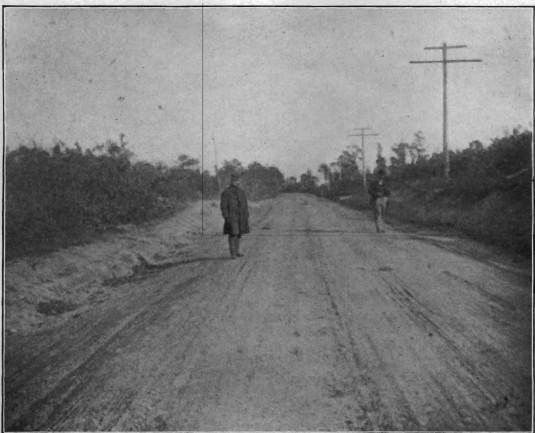
Little Egg Harbor Township County road, 1903, after improvement.
