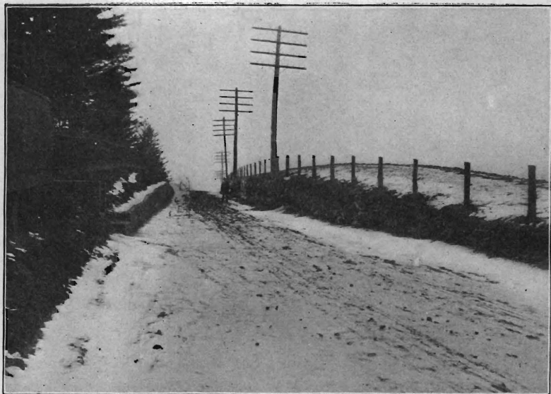
New Brunswick and Bound Brook road, Middlesex Co. Landing Hill, during improvement.
