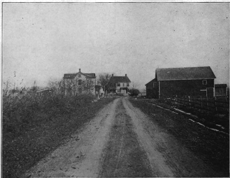
Neshanic road, Somerset Co., after improvement.
