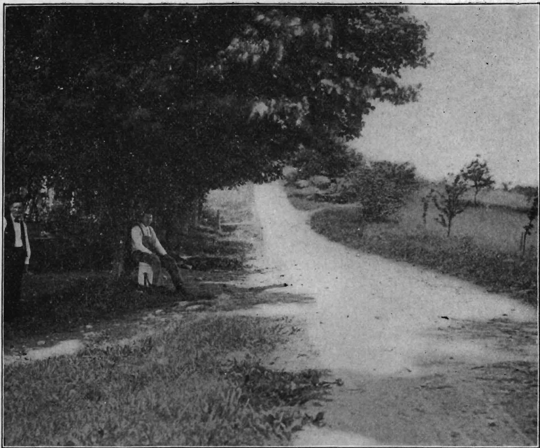
Squaw Brook road, Passaic Co., before improvement.
