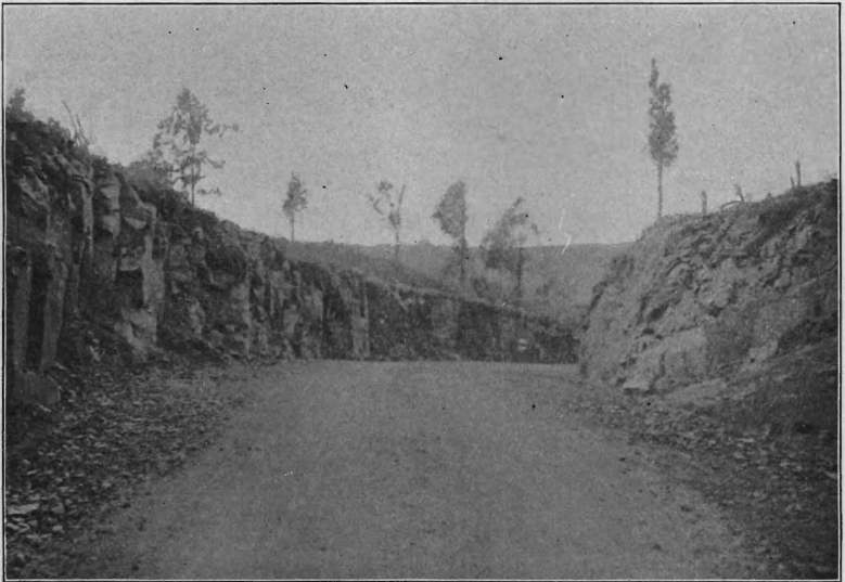
Marshall's Corner and Woodsville road, Mercer Co., showing 15-foot rock cut, after improvement
