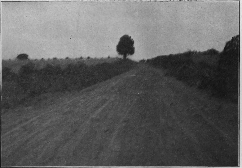
Stewartsville road, Warren Co., before improvement.
