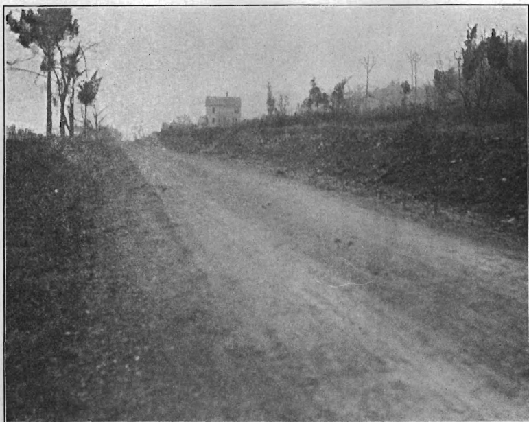
Clove road, Passaic Co., after improvement.
