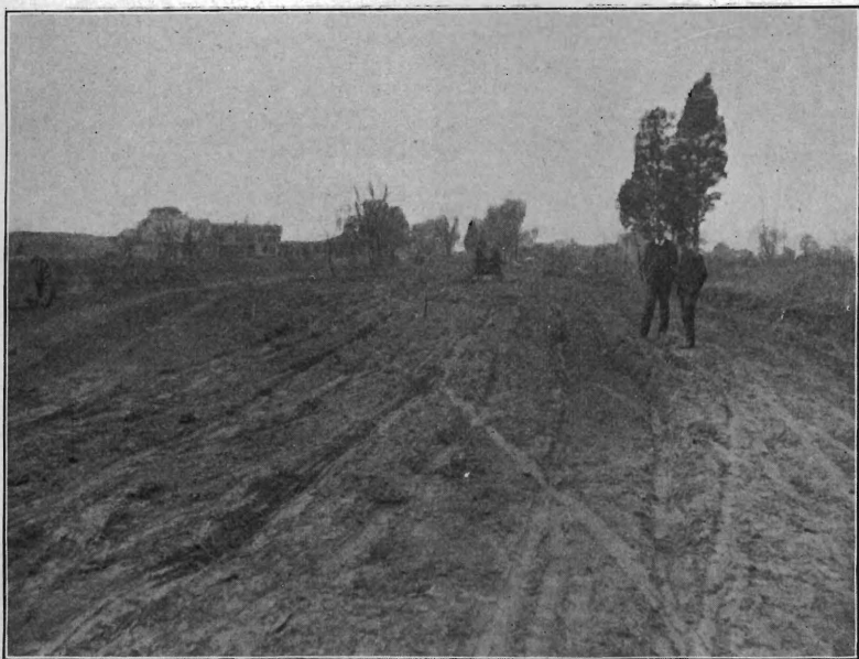
Sea Avenue, Point Pleasant, Ocean Co., before improvement.
