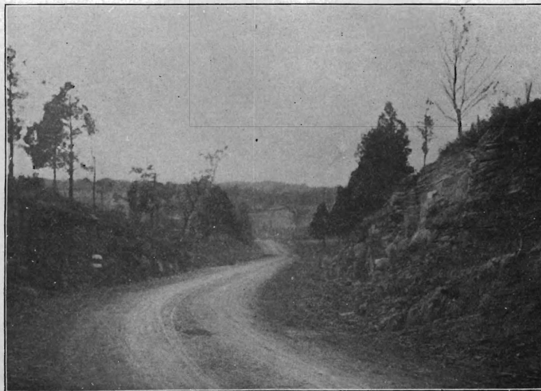
Marshall's Corner and Woodsville road, Mercer Co., after improvement.
