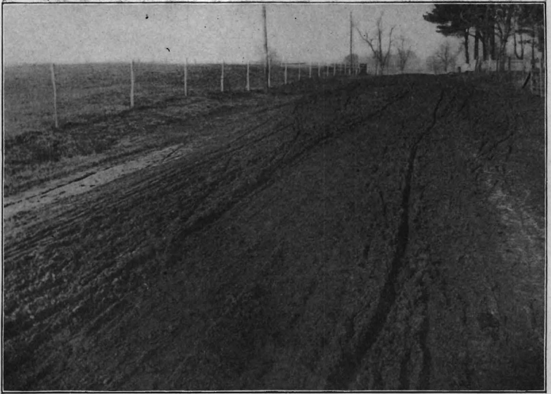
Manalapan and Freehold road, Monmouth Co., before improvement.
