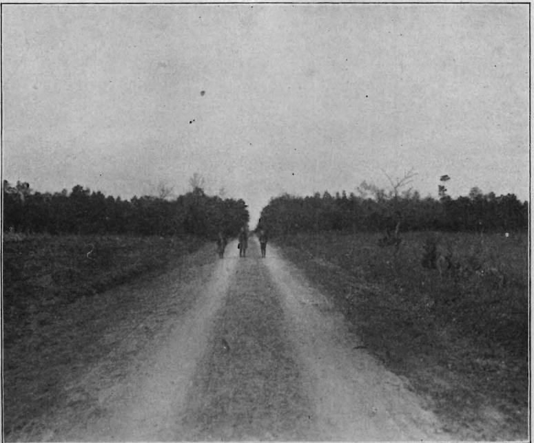
New Gretna road, Burlington Co., after improvement.
