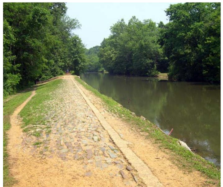
Delaware and Raritan Canal spillway at Kingston, Franklin Township, Somerset County. Spillways were built into the bank of a canal to allow excess water to spill out into adjacent waterways. *Photo by Z. Allen-Lafayette, 2004*
