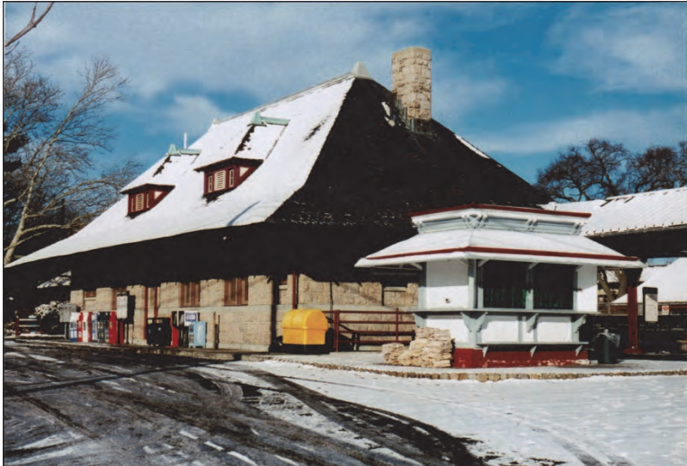
Fig. 16: Former Westfield CNJ station (now NJT), eastbound platform, and historic news kiosk. The station was built in 1912 and the photo was taken in 1997.
