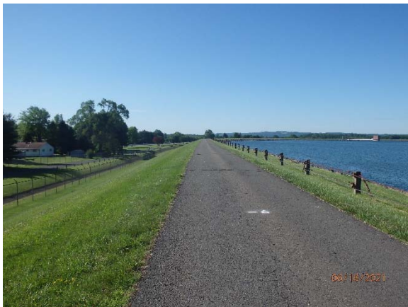
Spruce Run Reservoir Dam SE View From Sta. 5+50
