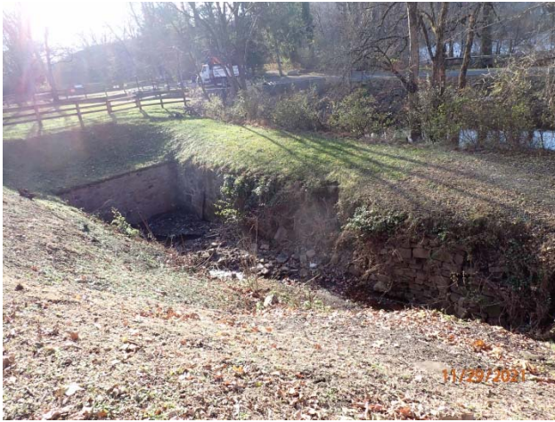
Existing condition of the Prallsville Culvert Pit.
