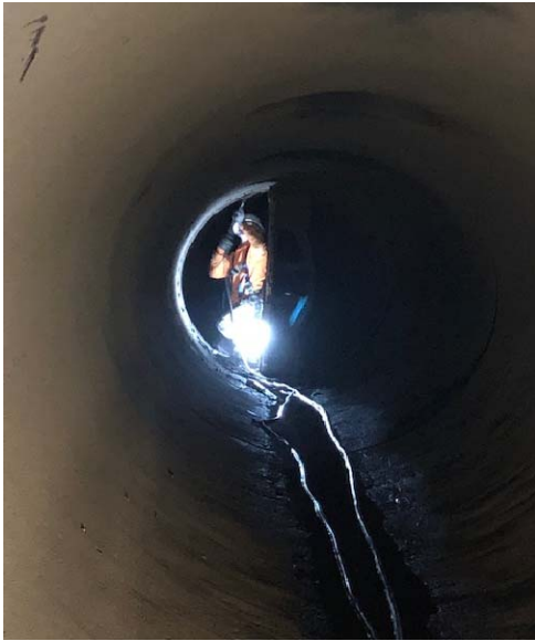
Transmission pipeline inspection and valve repair
