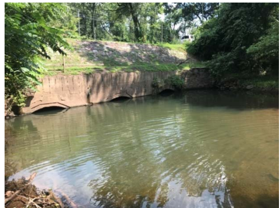
Six Mile Run Culvert (West Headwall)
