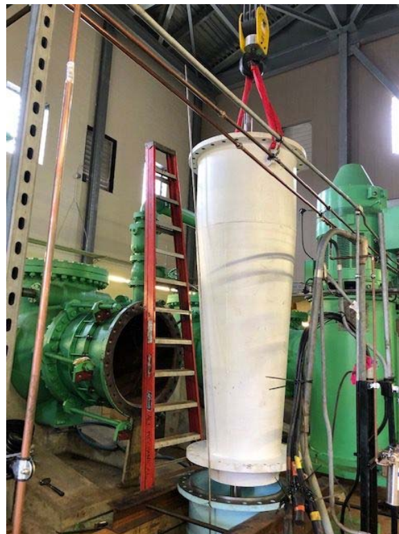
Reassembly of the intake pump
