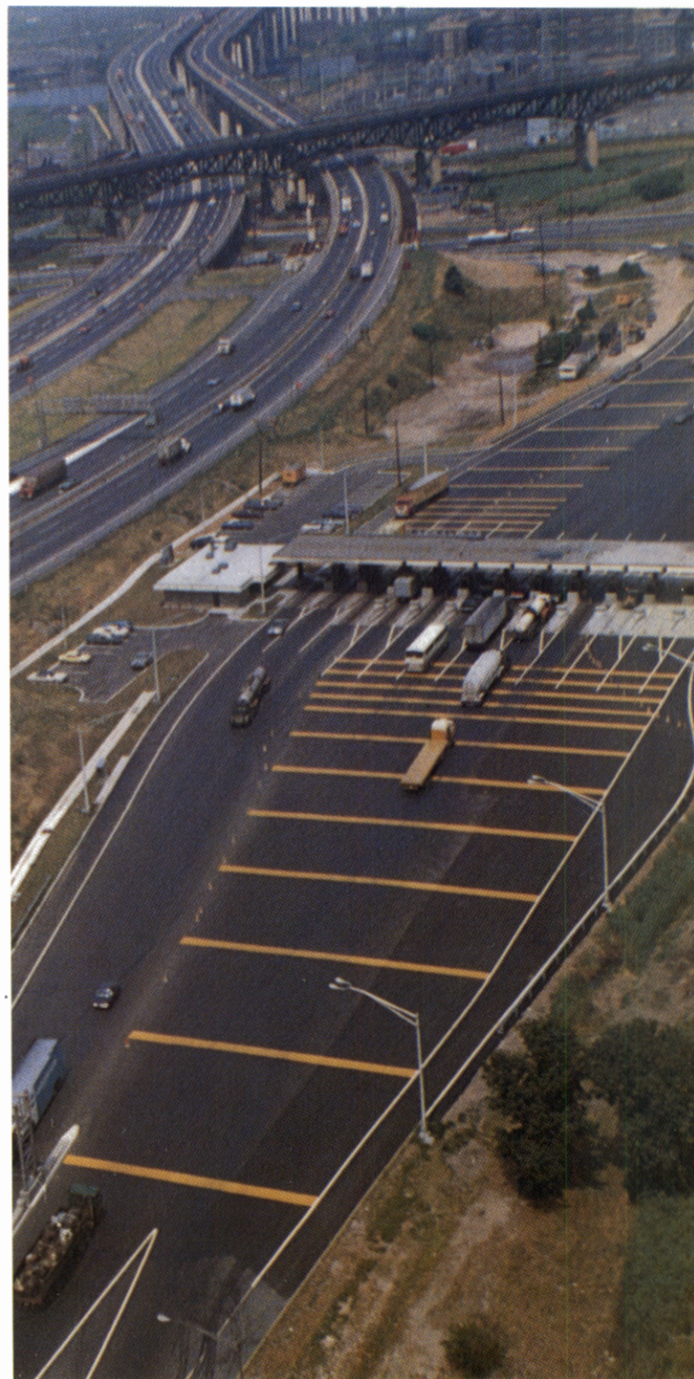
The mainline at Newark, with the Pulaski Skyway running above it and Route 1 below it. To accommodate traffic in this heavily industrialized area, Interchange 15E (at right) was expanded to 12 lanes and uniquely engineered to reduce costs.
