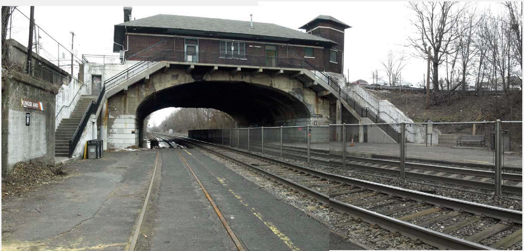
View of Kingsland Station from the low-level platform.
