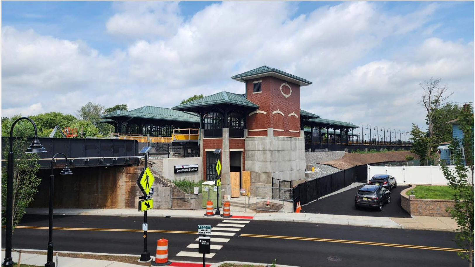
Outbound platform and elevator
