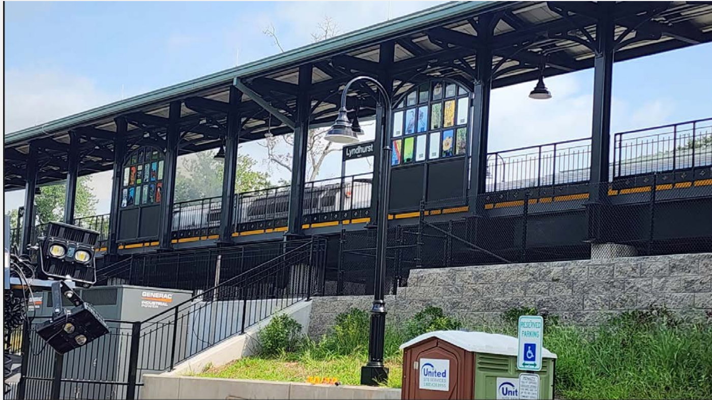
New high-level boarding platform (inbound)
