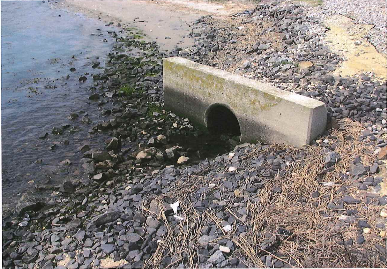
Storm water outfall in Atlantic City
