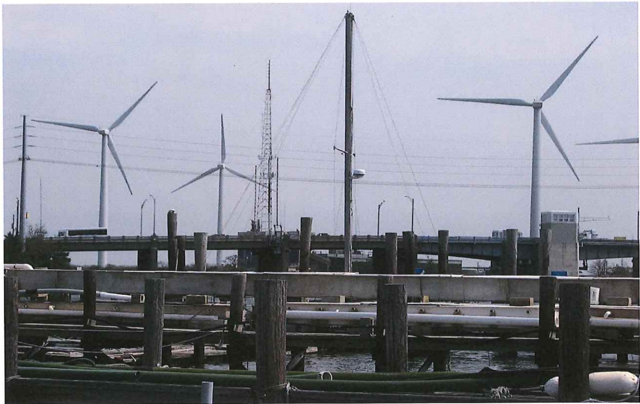
Wind turbines at Atlantic County Utilities Authority
