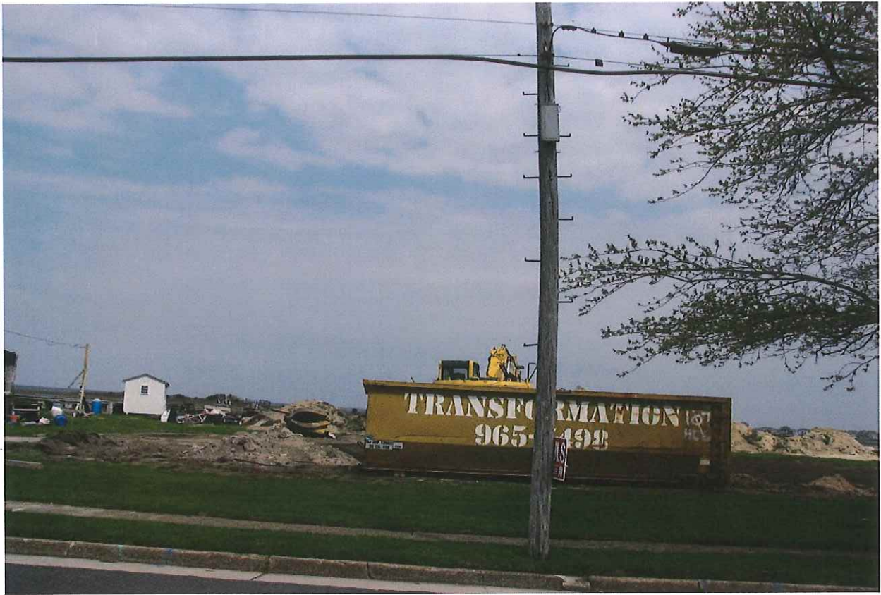
Rebuilding construction in Brigantine
