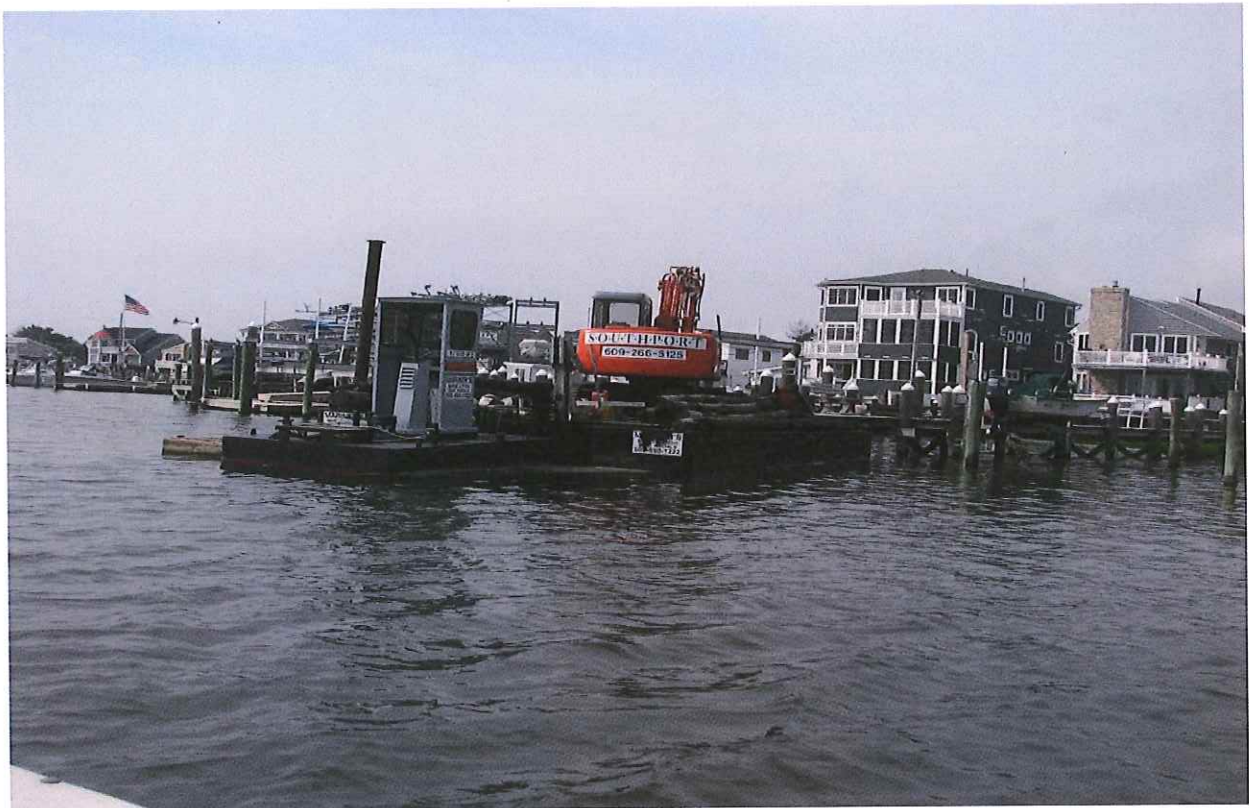
Rebuilding construction off of Brigantine
