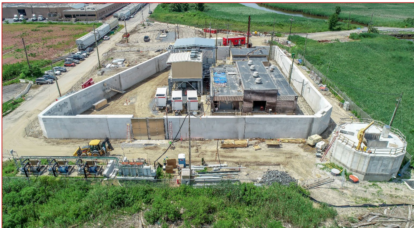
Restoration and Flood Mitigation
