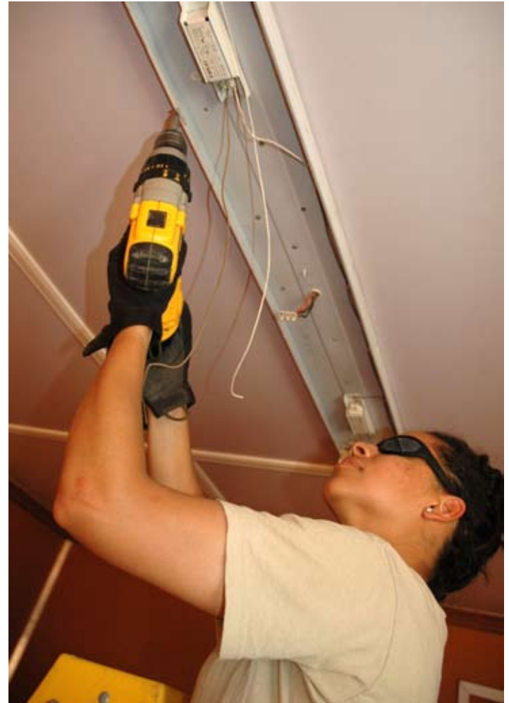
New Jersey Air Guard Staff Sgt. Anne McKenzie, an electrician, installs an overhead light fixture in a trailer her unit recently re-located at Baghdad International Airport. U.S. Air Force Photo by Master Sgt. Louis Conzo.
