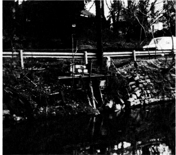
Condition of Route 29 wall in Ewing Township prior to repair.
