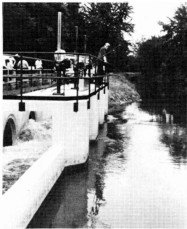
The new Scudders Falls Waste Gate structure in Ewing Township helps control flows in the Delaware and Raritan Canal.
