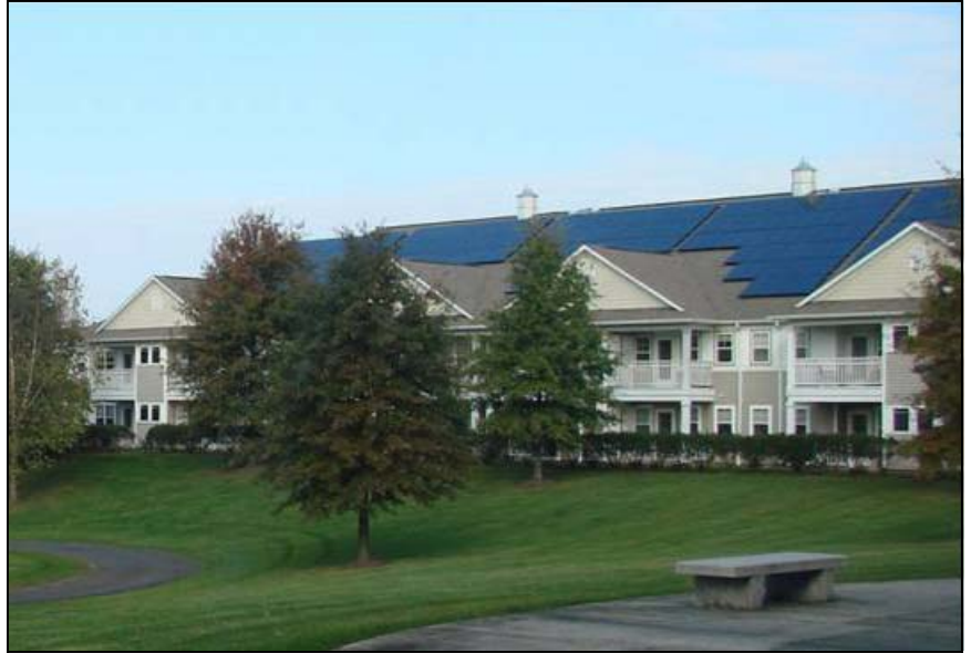
Absolutely Energized Solar Electric, Inc. , which benefited from EDA assistance in 2009, installed one of the largest pitched roof solar electric systems in New Jersey at Fellowship Village Retirement Community in Basking Ridge. Fellowship received a tax-exempt bond from the EDA to support the solar panel installation, which is expected to reduce 900,000 pounds of CO 2 each year.
