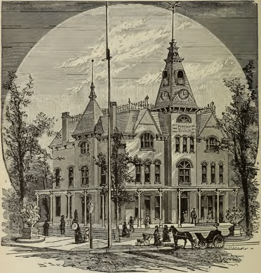
ASSOCIATION, TELEGRAPH AND POST OFFICE BUILDING.
