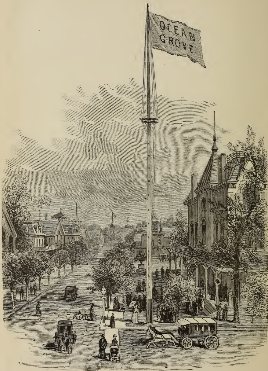
PILGRIM PATHWAY AND MAIN AVENUE, LOOKING TOWARDS THE AUDITORIUM.
