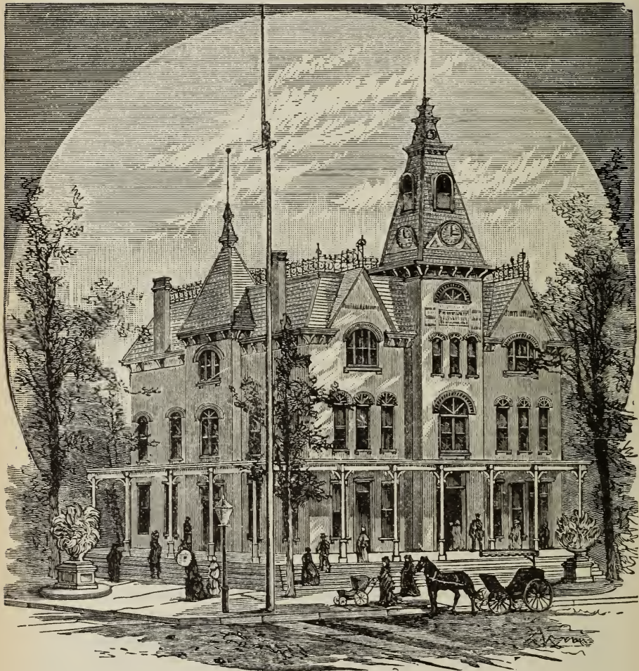
ASSOCIATION, TELEGRAPH AND POST OFFICE BUILDING.
