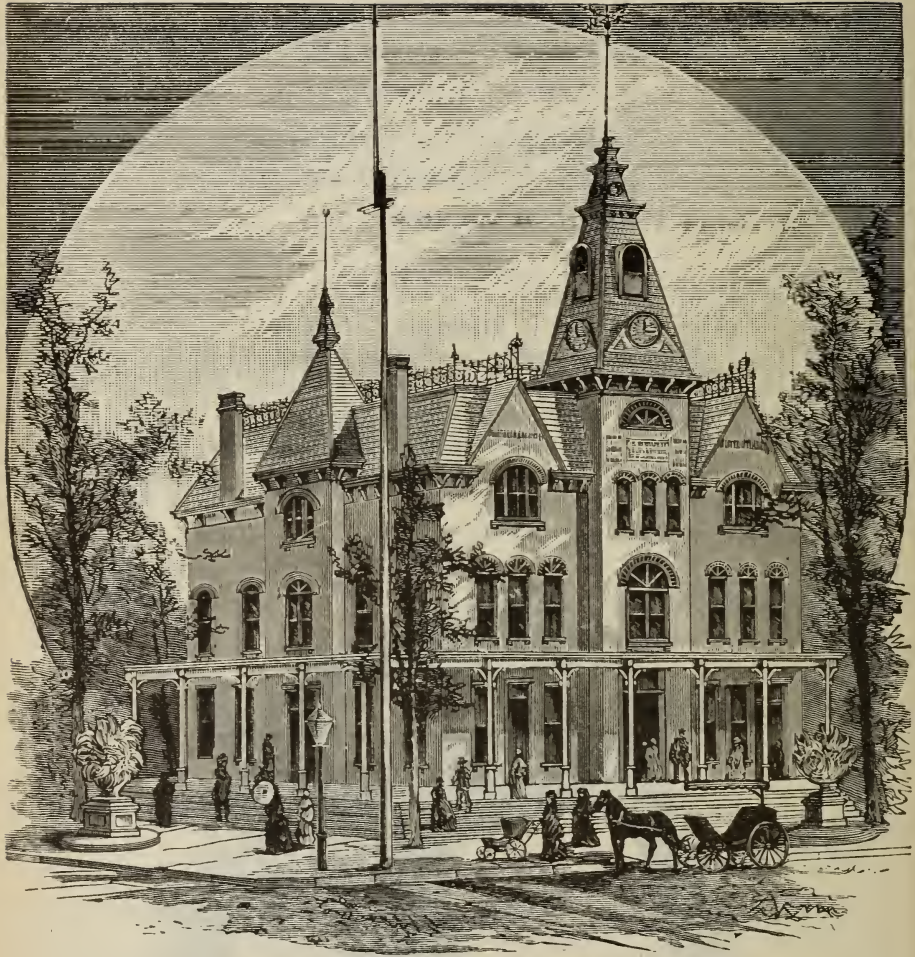
ASSOCIATION, TELEGRAPH AND POST OFFICE BUILDING,
