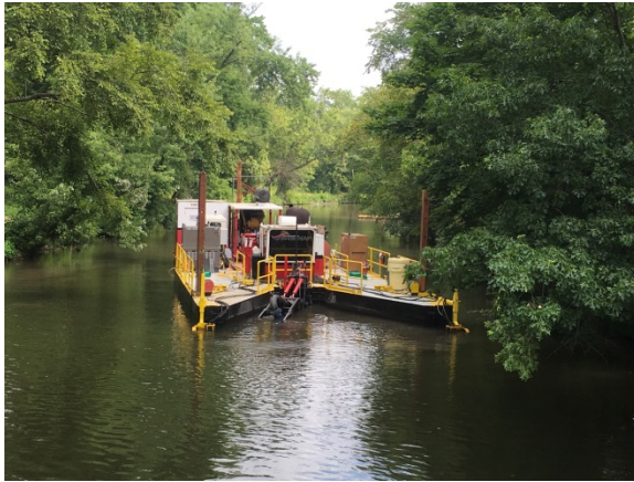
Photo shows one of three dredges currently in operation in July 2018. Note the boom extending into water in front of dredge in photo. Note three vertical square “spuds” keep equipment in place while dredging. Square plates at base of “spuds” prevent damage to clay liner at bottom of Canal. On-board computer and GPS maintain location and depth of boom and cutter head to prevent damage to the clay liner.
