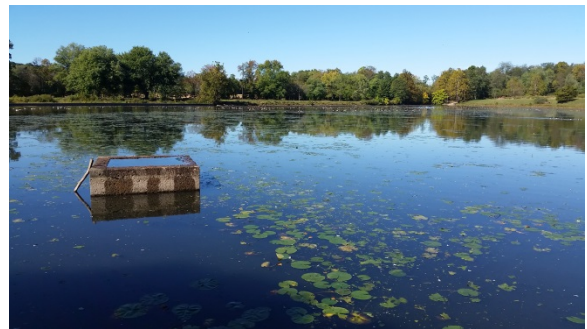
South Branch Pumping Station Intake Pond
