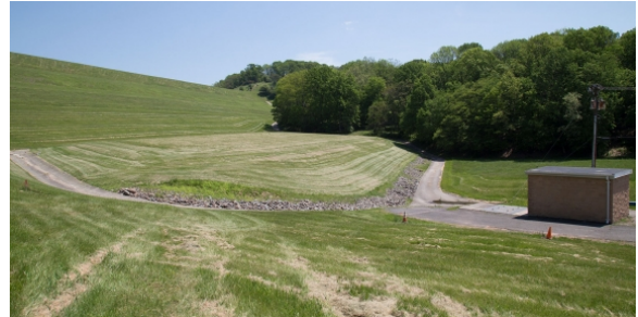
Round Valley South Dam and vault
