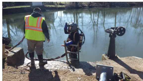
10-Mile Waste Gate was replaced “in the wet.” After flow through the gate was temporarily stopped on the river side of the structure, the gate was replaced without dewatering. In this photo, a diver enters the water to perform work on the replacement gates.
