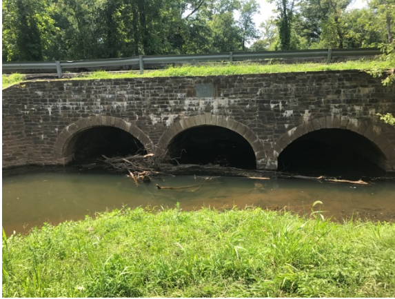
Upstream side of Six Mile Run Culvert.
