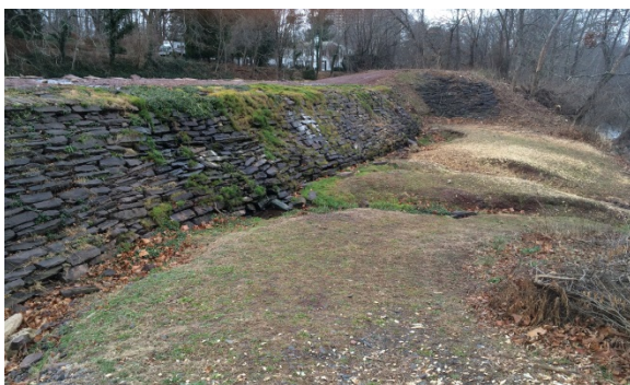
River side slope of Landing Lane Spillway.
