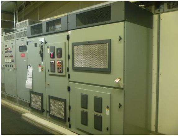
Variable speed controls for reservoir fill pump motors
