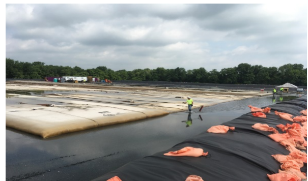
Geobags in constructed drying (staging) area during dredging operations. Silt-laden water is directed to the geobags that act like a filter. Clean (elutriate) water is discharged back to the Canal.
