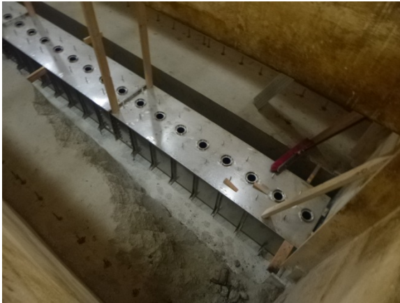
Underdrain reconstruction at the MWTP
