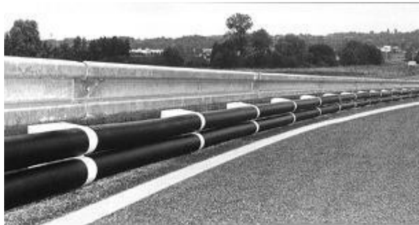
Figure 4. The Mototub by Sodirel. The Mototub is made from 70% recycled material and prevents motorcyclists from hitting the posts of the guardrail [30].
