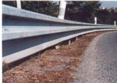
Figure 3. The Plastrail by Solidor. This plastic covering provides protection to motorcyclists by covering the posts of the guardrail [31].
