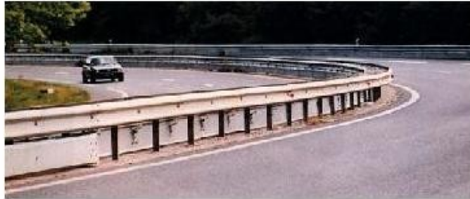
Figure 2. Metal shield developed by SEC-Envel. The flexible metal covers the hazardous posts and prevents motorcyclists from colliding with them [30][30] (left) and [31] (right).
