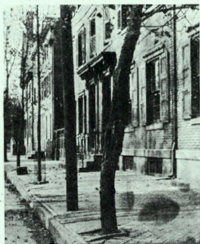
NO GUARD—ALL PAVEMENT Give your trees protection and a place to grow
