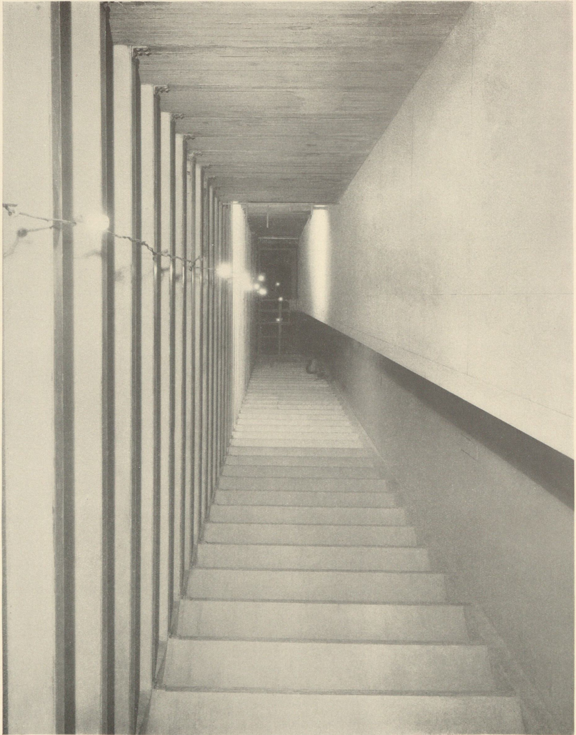
FRANKLIN SQUARE STATION, PHILADELPHIA HIGH-SPEED LINE
