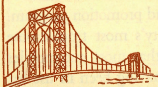
GEO. WASHINGTON BRIDGE
