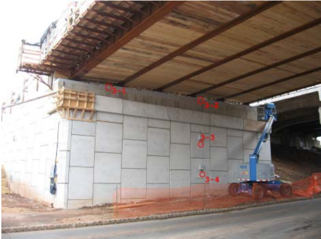
Figure 15. Optical Prism Locations at Wall 3
