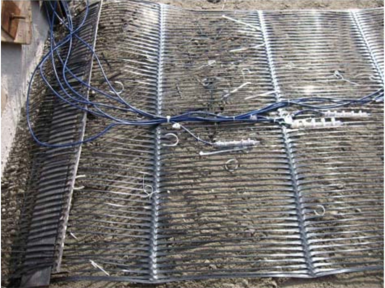
Figure 21. Instrumented Geogrid with Strain Gages
