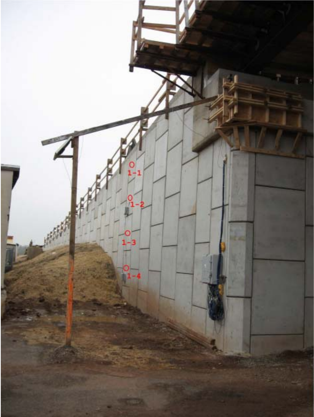
Figure 14. Optical Prism Locations at Wall 1
