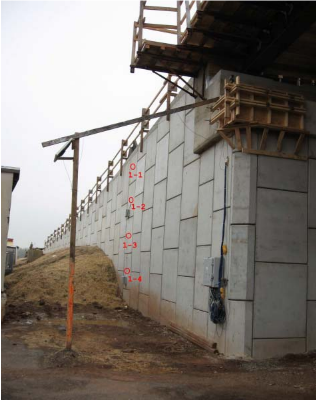
Figure 35. Wall 1 Survey Point Locations
