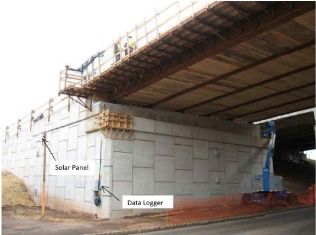
Figure 23. Wall 1 and Wall 3 at End of Construction
