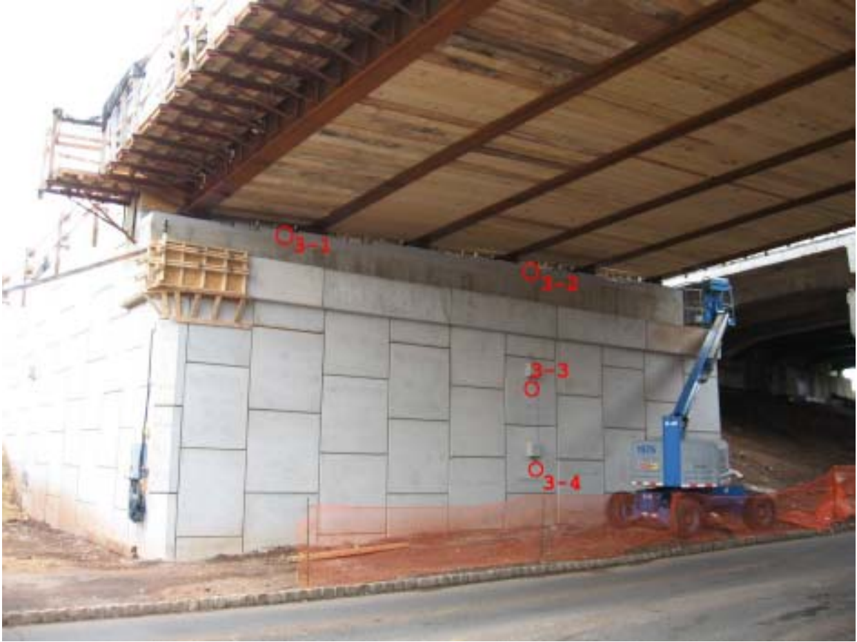
Figure 36. Wall 3 Survey Point Locations
