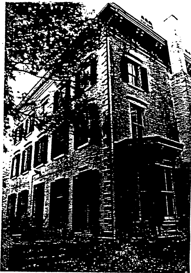
0233-31 East facade, from the north corner. View to southwest. Neg. file # 19847-18
