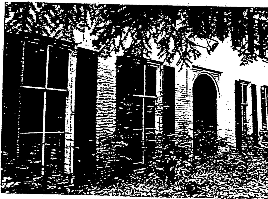
0233-31 East facade, first story. Entrance at center. View to northwest. Neg. file # 19847-17
