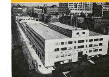
NEW YORK UNION MOTOR TRUCK TERMINAL
