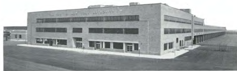
The Newark Truck Terminal, largest in the world, was readied in 1955 for commercial trucking operations.
