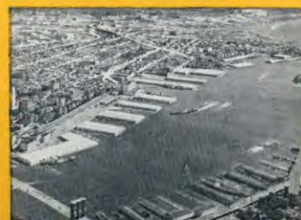
BROOKLYN-PORT AUTHORITY PIERS
