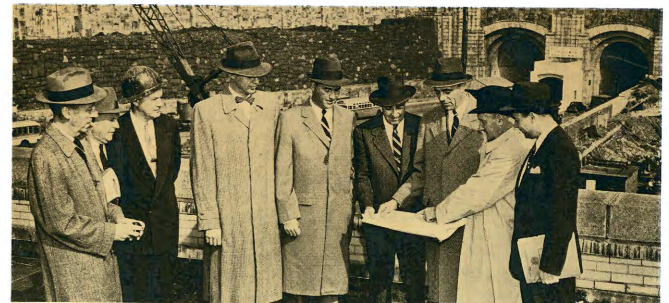
New Commissioners, James C. Kellogg, III (fifth right) and Thorn Lord (third right), during an inspection of the Lincoln Tunnel, are briefed on details of construction of that arterial crossing's $100,000,000 Third Tube by Assistant Executive Director Matthias E. Lukens (fourth right) and other members of the Port Authority staff.
