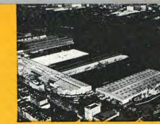
HOBOKEN-PORT AUTHORITY PIERS
