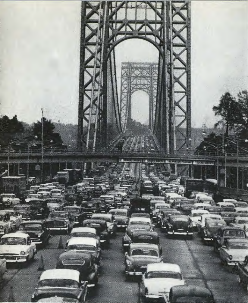
The year's peak traffic often produced demands beyond the capacity of the George Washington Bridge, here shown during busy Labor Day weekend. Addition of a proposed second level to this busy crossing would provide increased capacity to handle ever increasing needs of interstate vehicular travel.
