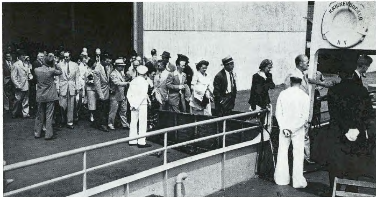
After inspecting Pier C at the Hoboken-Port Authority Piers, New Jersey Legislators and their families board the ship on which they will continue their sixth annual inspection of the New Jersey-New York Port and of the Port Authority's facilities.
