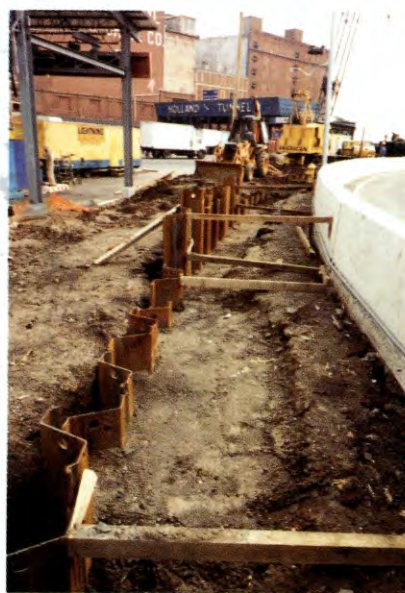
Major work continued during the year to rebuild and expand the Holland Tunnel's Jersey City entrance roadway area and toll plaza.
