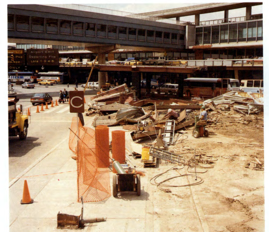
LaGuardia Airport redevelopment in 1989 included work on roadways, infrastructure and utility relocation.
