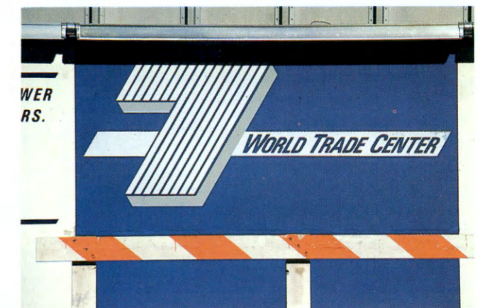
Construction got under way for the World Trade Center's final structure, Seven World Trade Center, scheduled to open in 1987.
