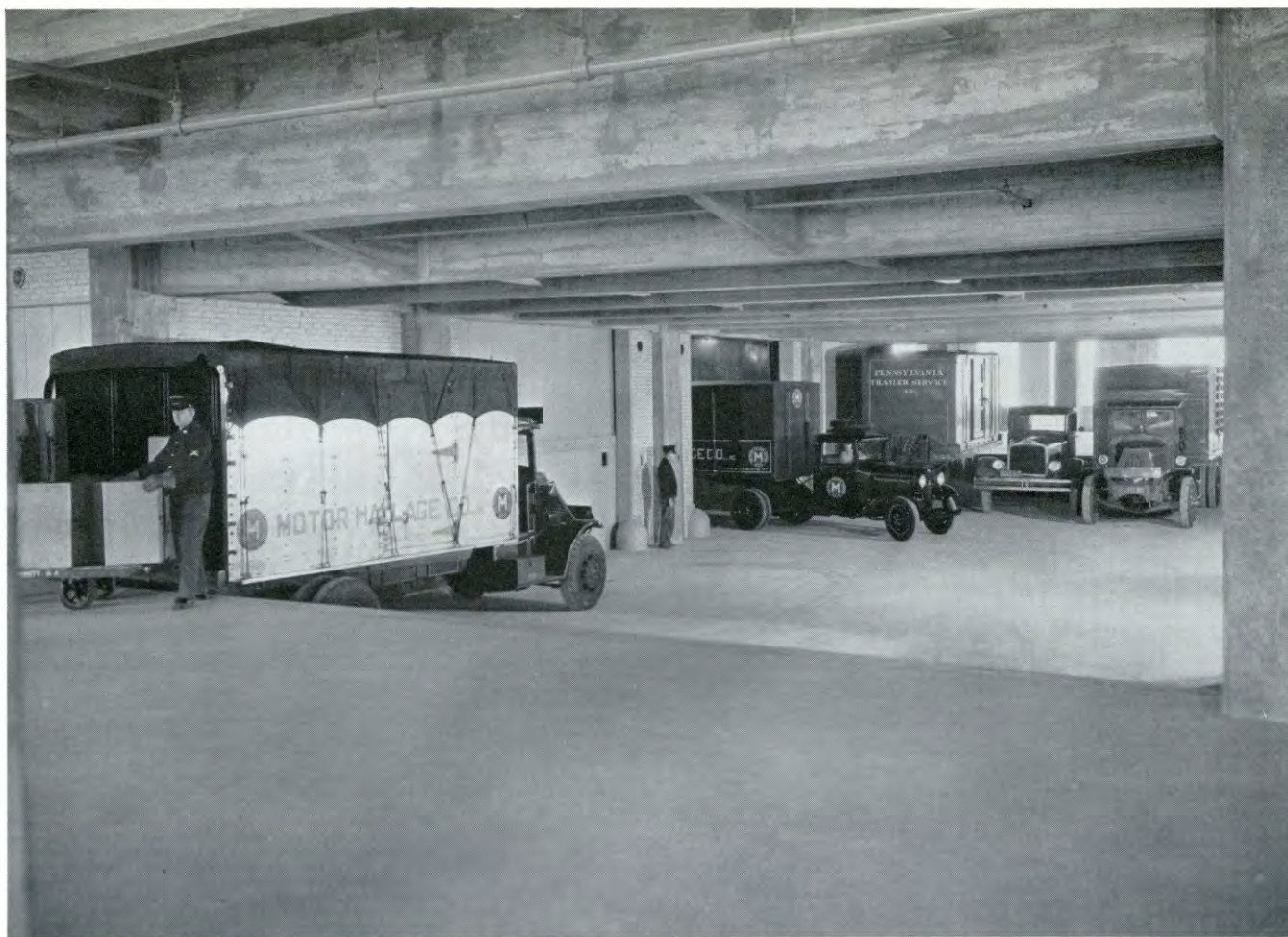
Valuable Short Cut in Distribution—Street Level Convenience in Freight and Parcel Handling is Afforded Upper Floor Tenants of Port Authority Commerce Building.
