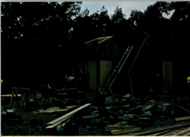
Beautiful new sanitary facility at Sunrise Mountain nears completion.
