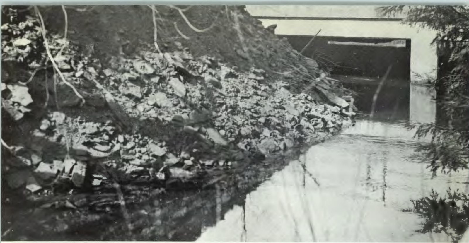
Another type of encroachment violation
