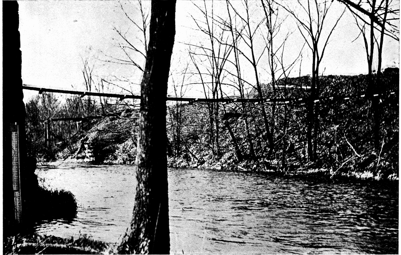
Fig. 2. Stream gaging station on Pequest River at Pequest Furnace, showing staff gage and foot bridge for making discharge measurements. (p. 72)
