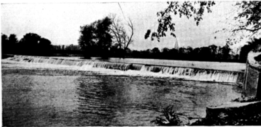
Fig. 11. Oradell dam on Hackensack River—water supply reservoir. (p. 58)
