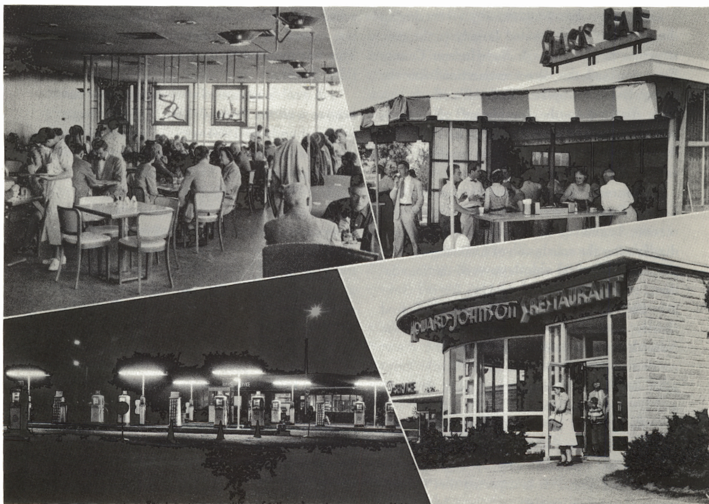
Typical service area
