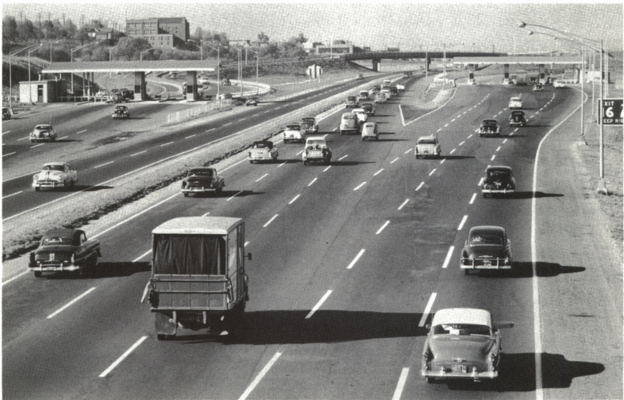
View of activity at Lincoln Tunnel interchange
