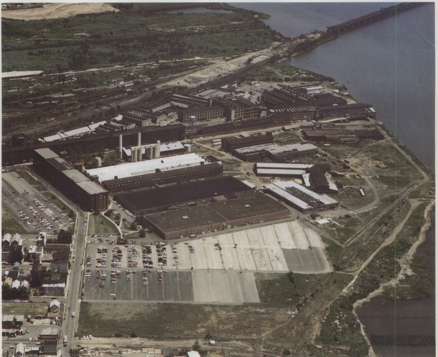
Seaport Industrial Center as it presently exists.
