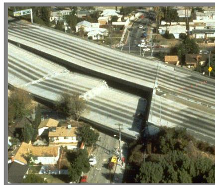
Bridge damage from the 1994 earthquake in Northridge, CA
