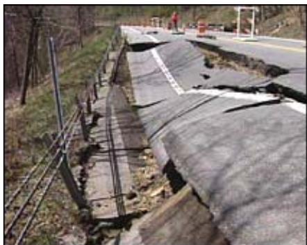
Embankment damage from the 2001 Plattsburg earthquake in NY State
