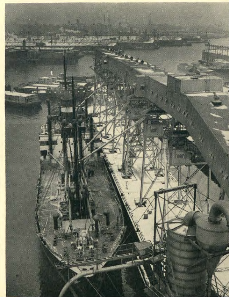
New loading gallery in operation at Grain Elevator delivering a full cargo of Government-owned wheat to the SS Pierre de Saurel. Previous to the installation of this gallery, grain from the elevator required delivery to ocean vessel by lighters and transfer by floating elevators. The new gallery eliminates the need for the lighterage service and results in an average saving to the shipper of 1 3/4 cents per bushel.
