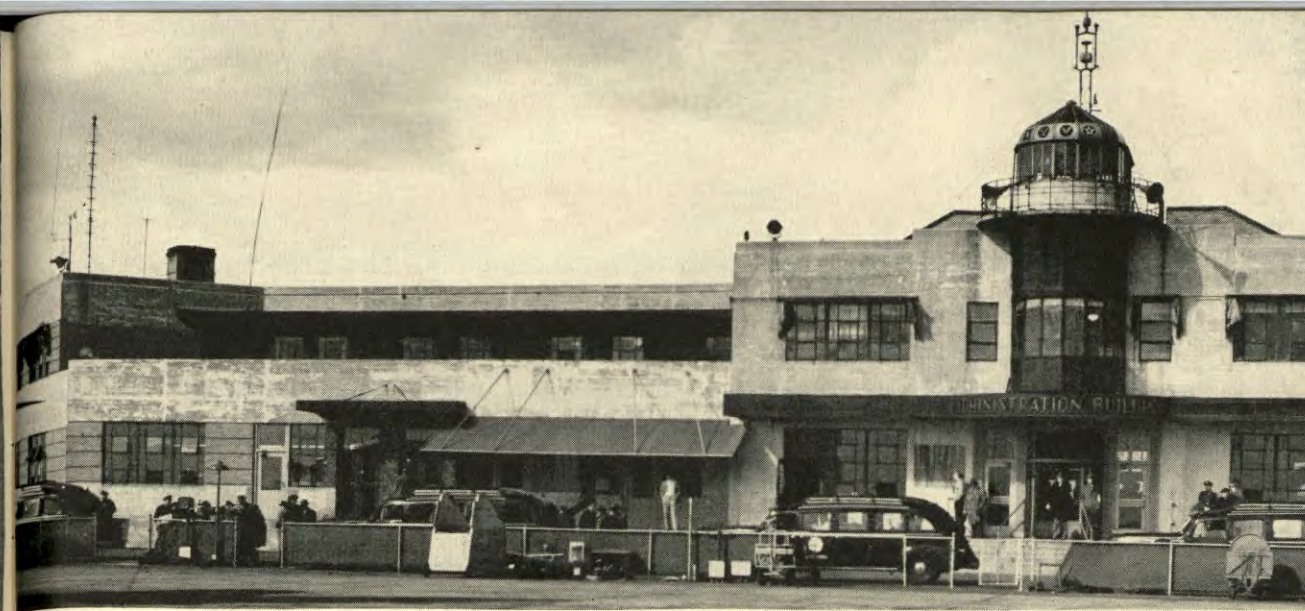
The present terminal building at Newark Airport which the Port Authority will replace with a great terminal structure.
