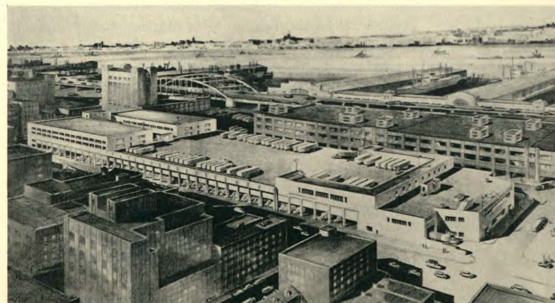
Sketch of the $9,000,000 New York Union Motor Truck Terminal under construction near the Holland Tunnel. This three-block-long "post office" for truck freight will reduce traffic congestion on Manhattan streets and along the waterfront.
