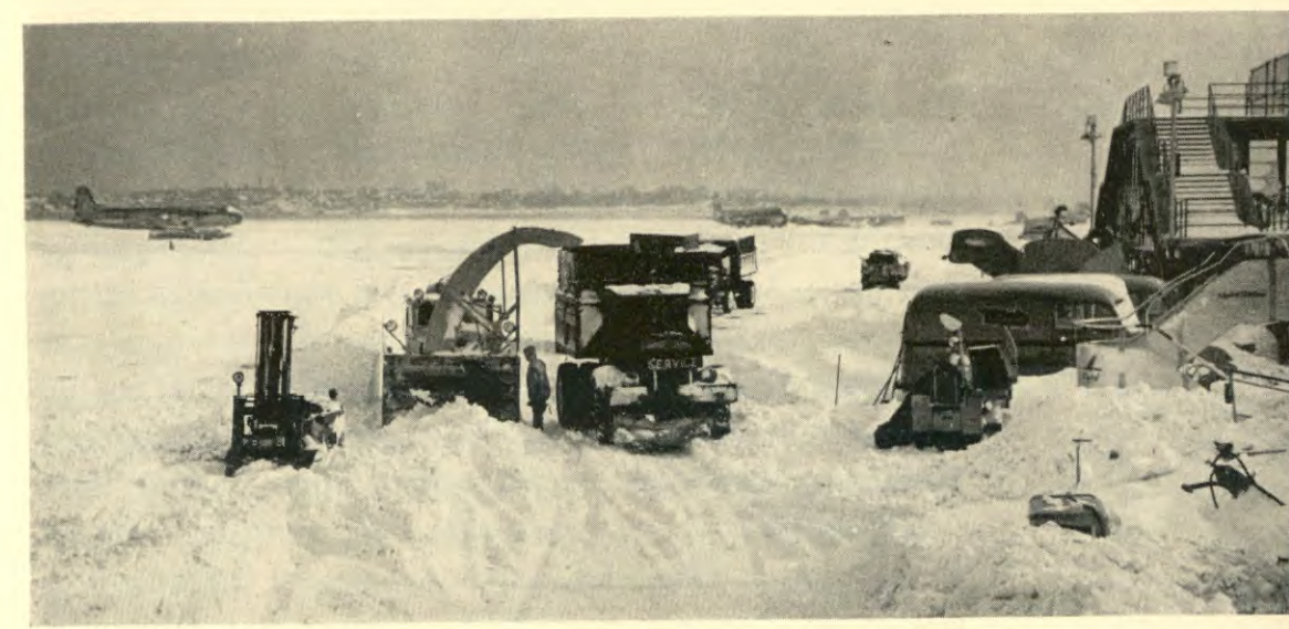
Snow-eaters loading moving trucks with snow on the ramp area during the Big Snow of 1947.
