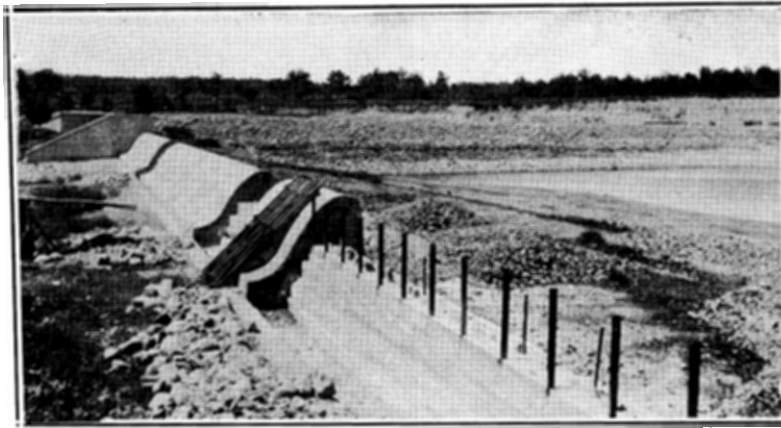
Fig. 10. Raising dam at Oak Ridge Reservoir, on Pequannock River—Newark Water-Supply System.
