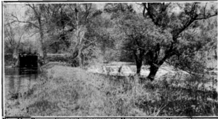
Fig. 11. Power dam and raceway on Musconetcong River, above Riegelsville.
