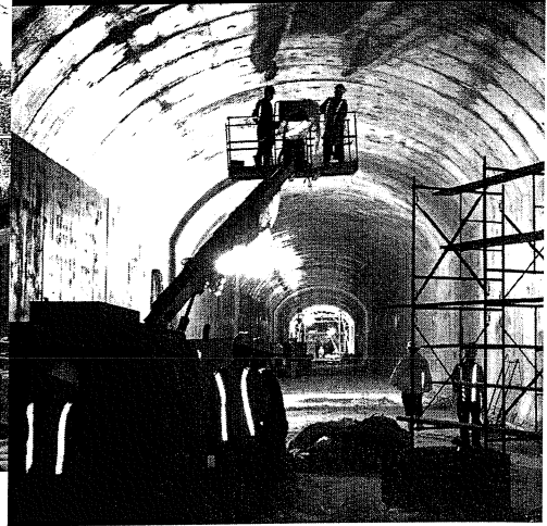
Bergen Tunnel north tube
