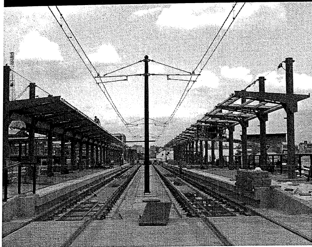
HBLR construction at Hoboken
