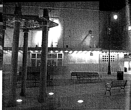
Raymond Plaza Improvements/ Market Street Bus Lane, Newark Penn Station
