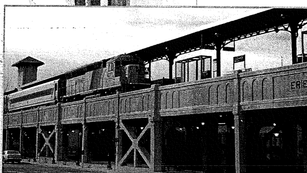
Paterson Station viaduct
