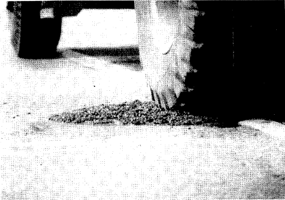
Figure 7. Throw-and-Roll Repair Method: Compaction of Material Using the Wheels of a Truck on Site (5)
