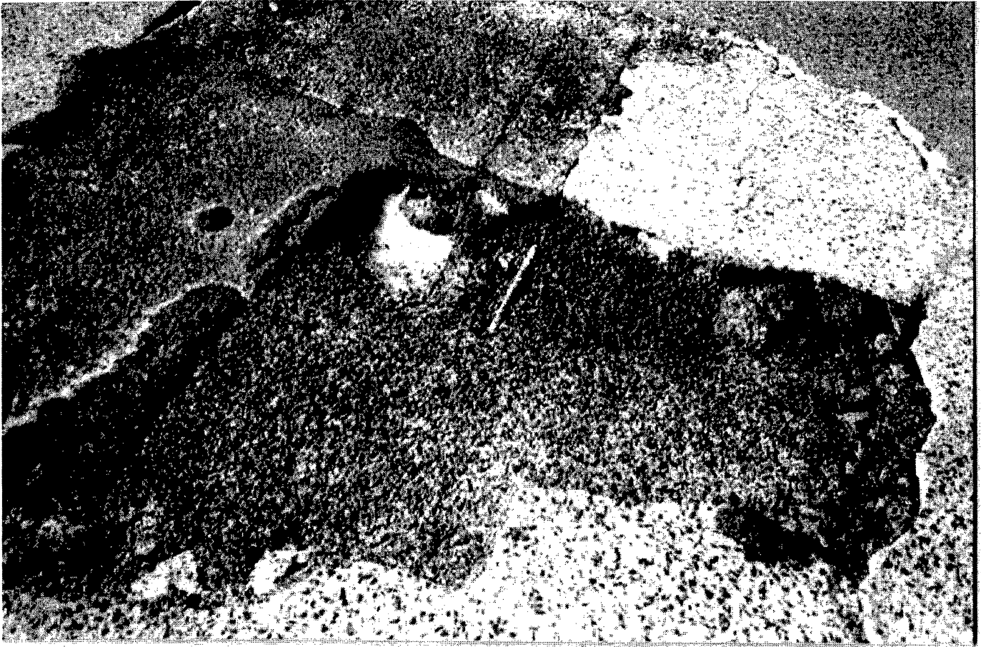
Figure 42. Permapatch 2 Month Inspection, #1 Rt. 21 NB Passaic, #2 Rt. 1&9 NB MP 49.5 Passaic
