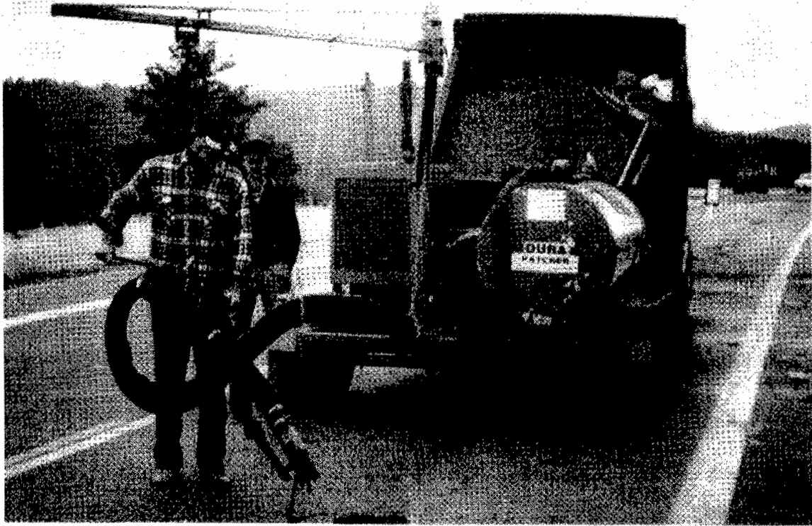
Figure 10. Spray Injection Method of Pothole Repair (5)
