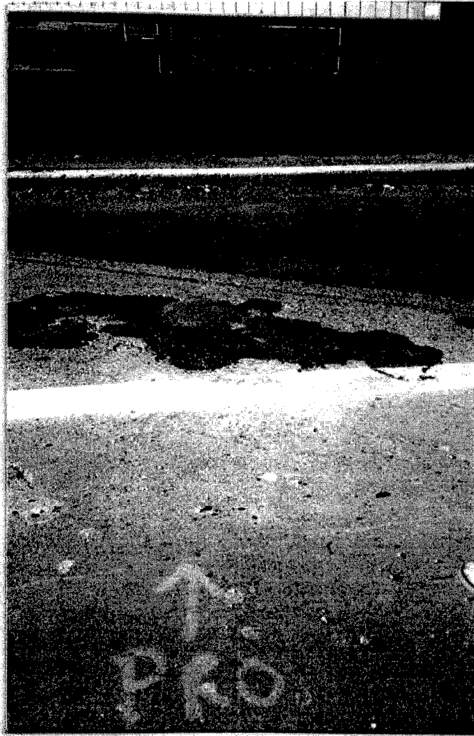
Figure 60. Wespro 2 Month Inspection, Rt. 21 SB MP 12.36 Passaic
