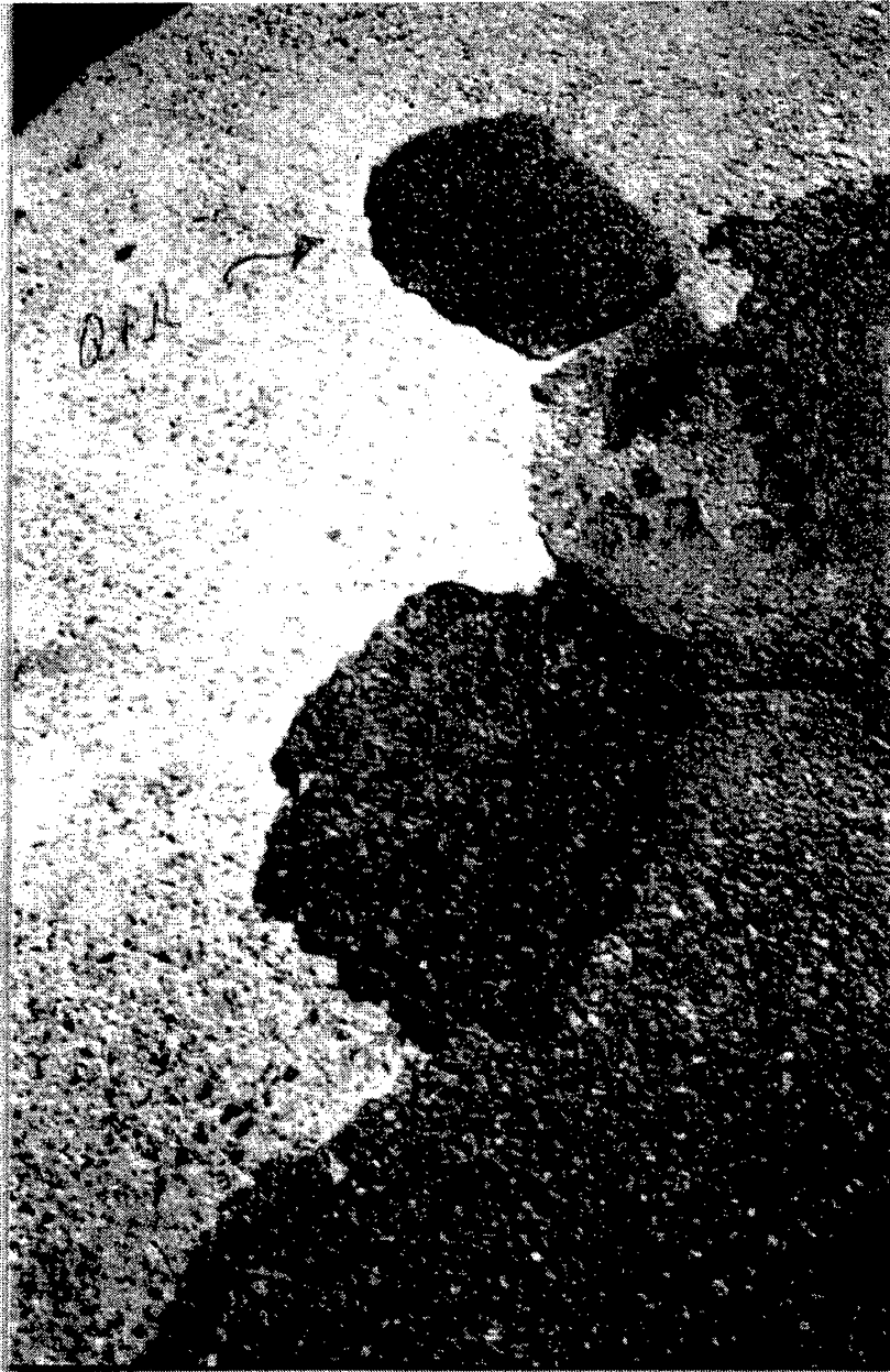
Figure 44. QPR 2 Month Inspection, Rt 21 SB MP 12.0 Passaic
