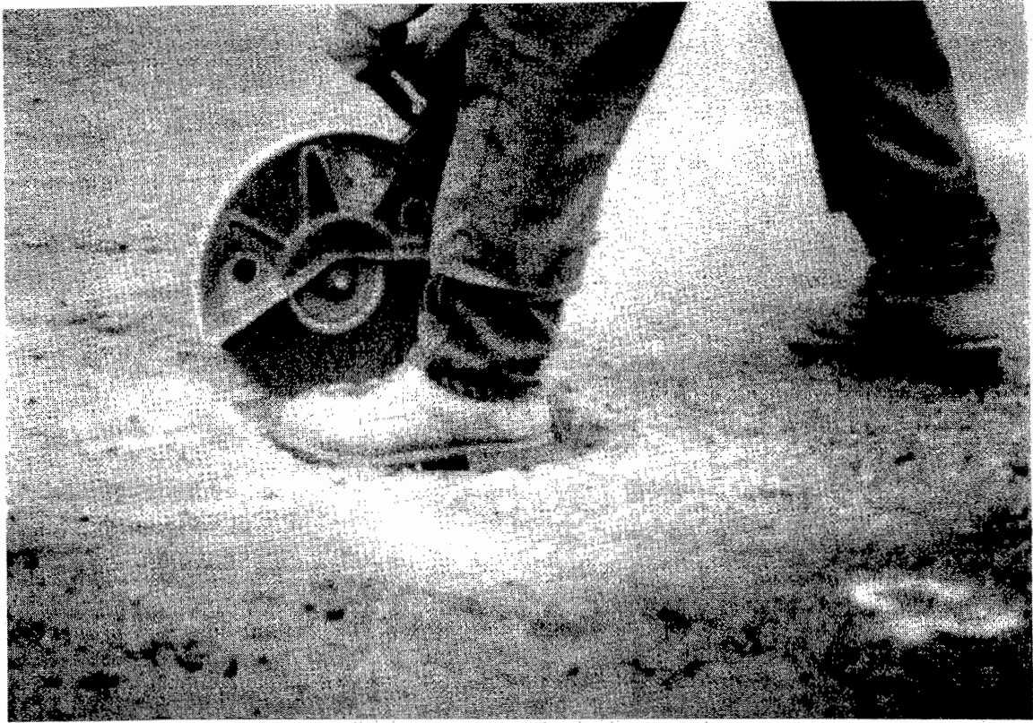
Figure 8. Semi-permanent Method of Pothole Repair: Saw-Cutting of Edges (5)
