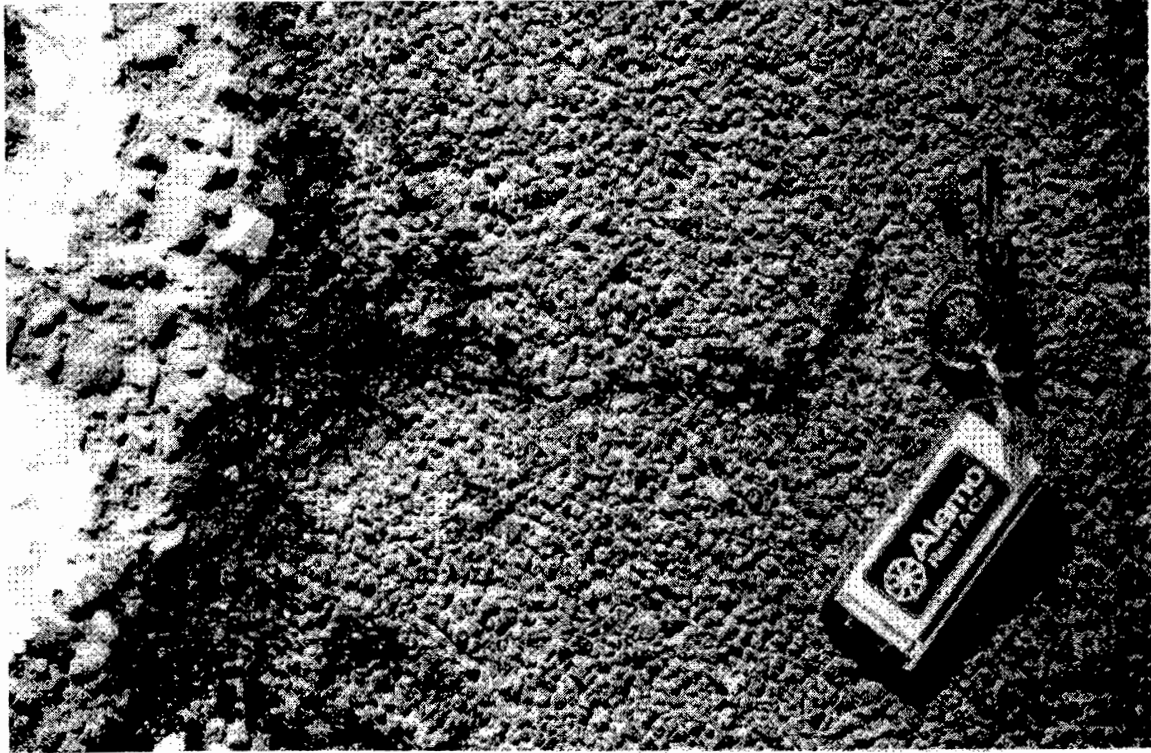
Figure 2. Cracking Distress (3)
