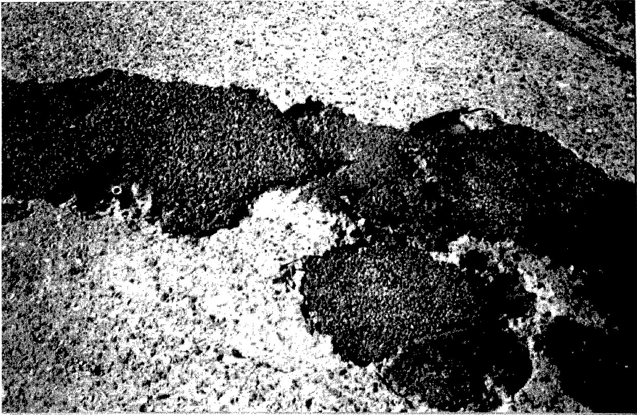
Figure 43. QPR 2 Month Inspection, Rt. 21 SB MP 12.0 Passaic
