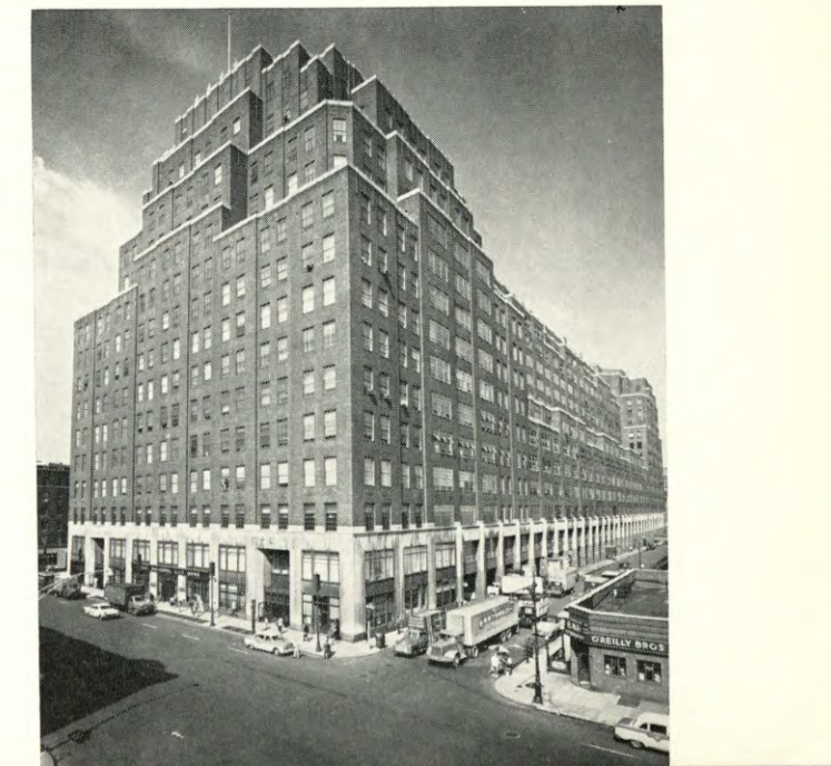
The Port Authority Building handles freight for five railroads and is a major merchandise handling station in Manhattan.
