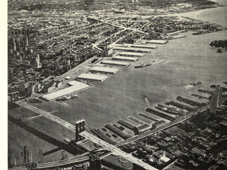
Construction at the Brooklyn-Port Authority Piers, shown in this artist's rendering, reached the half-way mark in 1959 with the completion of the fifth new pier. Piers 1, 2 and 3, the three piers in the foreground, are in operation. (See pages 16-17)
