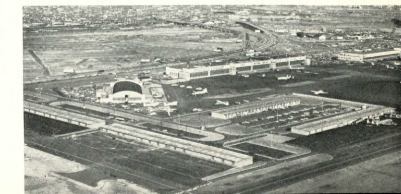
The new, four-building air cargo center (foreground) at Newark Airport was dedicated on December 2, 1959. The center will facilitate the movement of air cargoes through Newark Airport.
