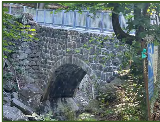
Figure 20: The Arch Bridge 5
