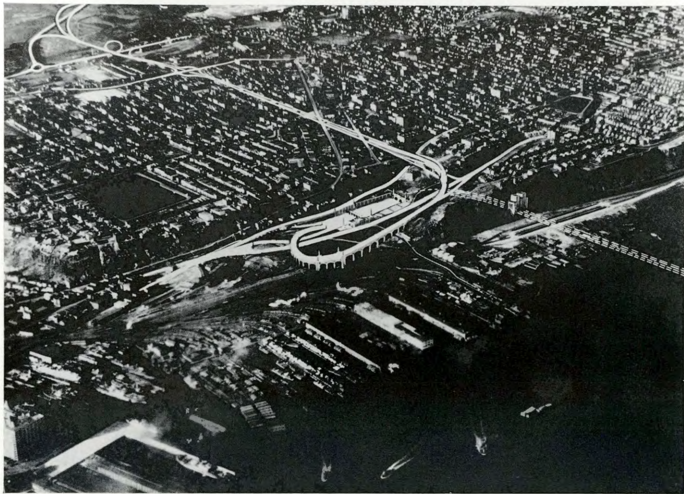
Midtown Hudson Tunnel—Aerial View Showing Graphic Ultimate Approach Plan in New Jersey
