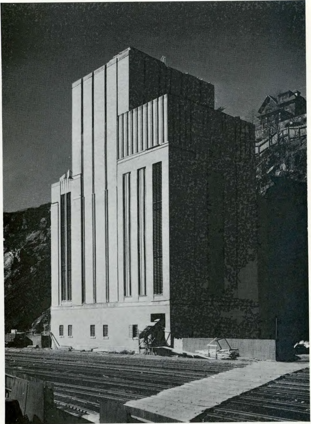
Midtown Hudson Tunnel—New Jersey Ventilation Building
