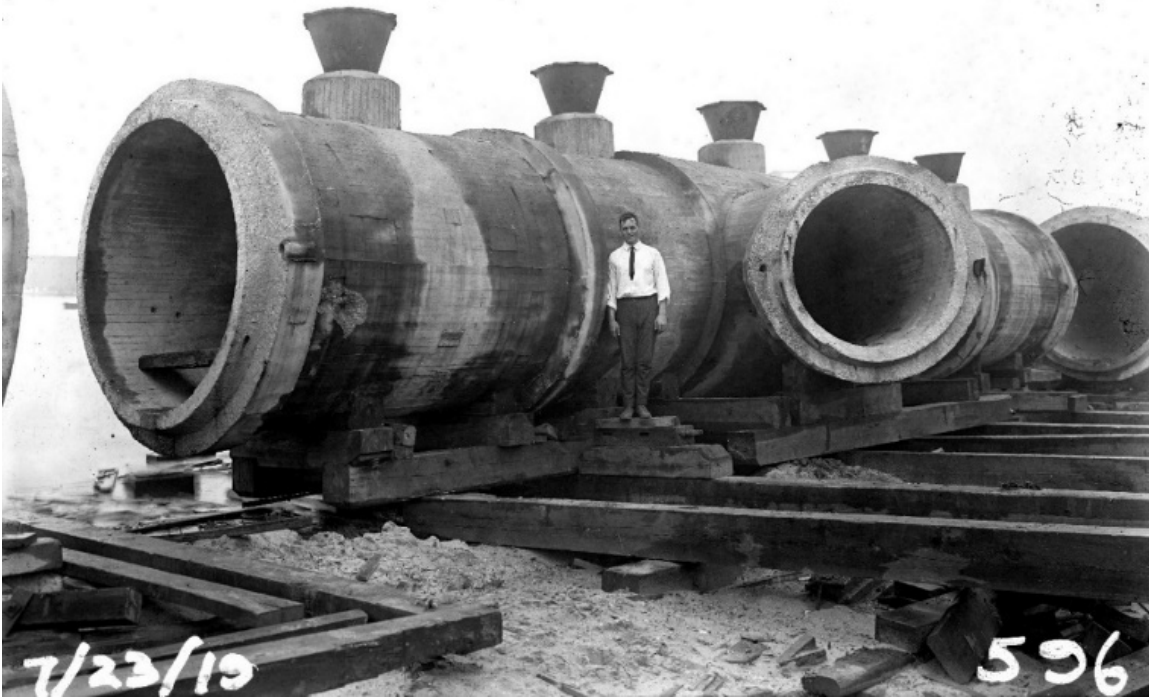
Figure 35. Concrete outfall pipes of the PVSC system. Source: Passaic Valley Sewerage Commission, Construction of outfall pipe, 1920s . https://nj.gov/pvsc/who/history/photos/images/plant/img020.jpg
