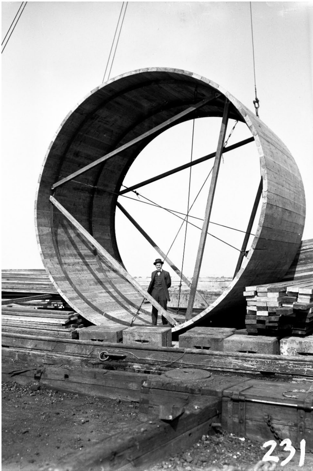
Figure 36. Wooden frame for the construction of a PVSC outfall pipe. Source: Passaic Valley Sewerage Commission, Construction of outfall pipe, 1920s. https://nj.gov/pvsc/who/history/photos/images/plant/img148.jpg
