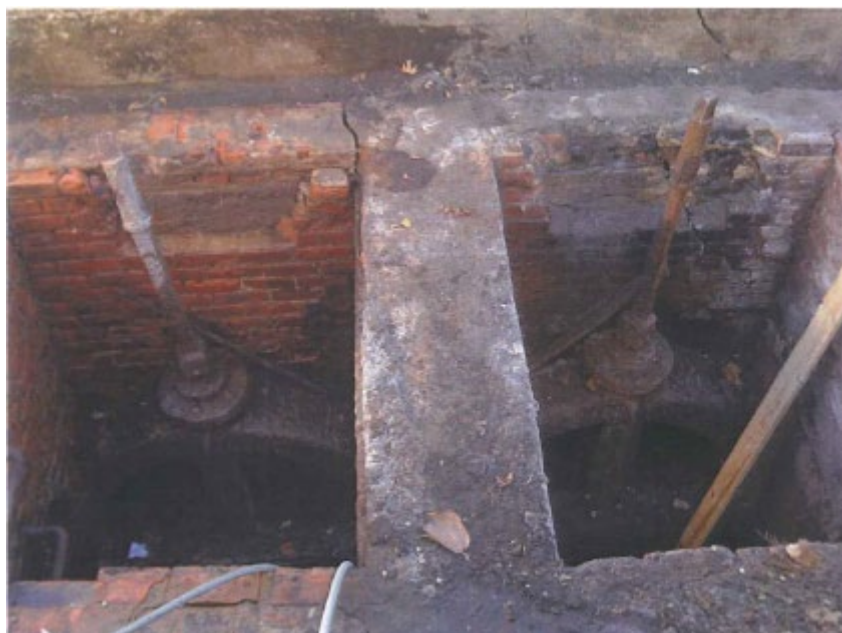
Figure 68. Brick tidal gate with iron mechanisms in the Observer Highway sewer.
