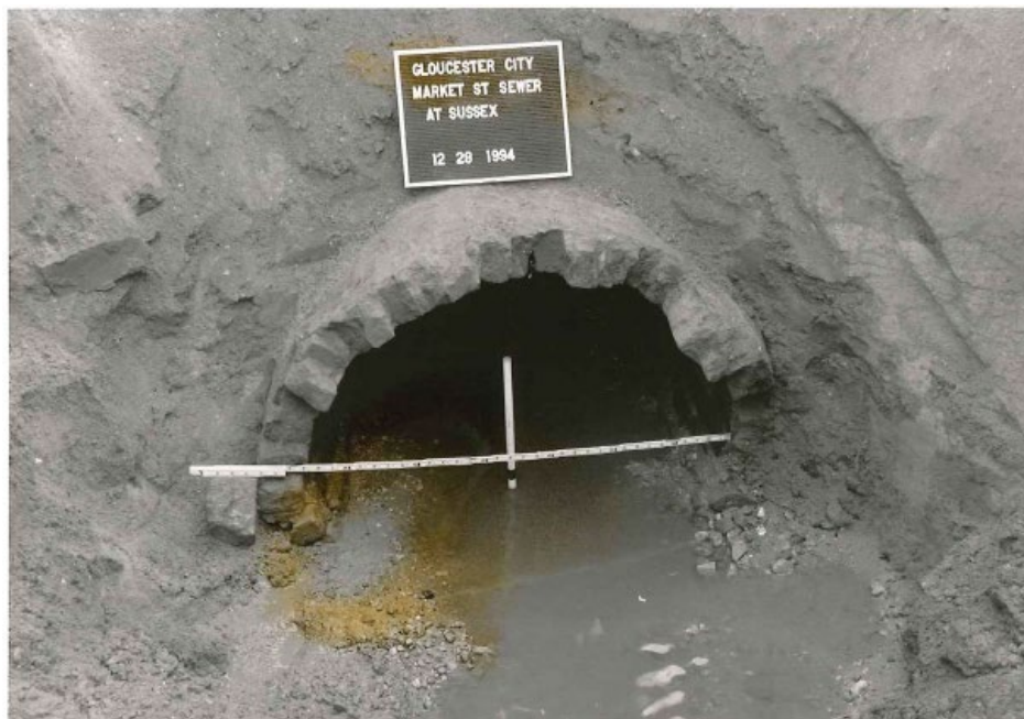
Figure 50. Photograph of the Market Street brick sewer.
