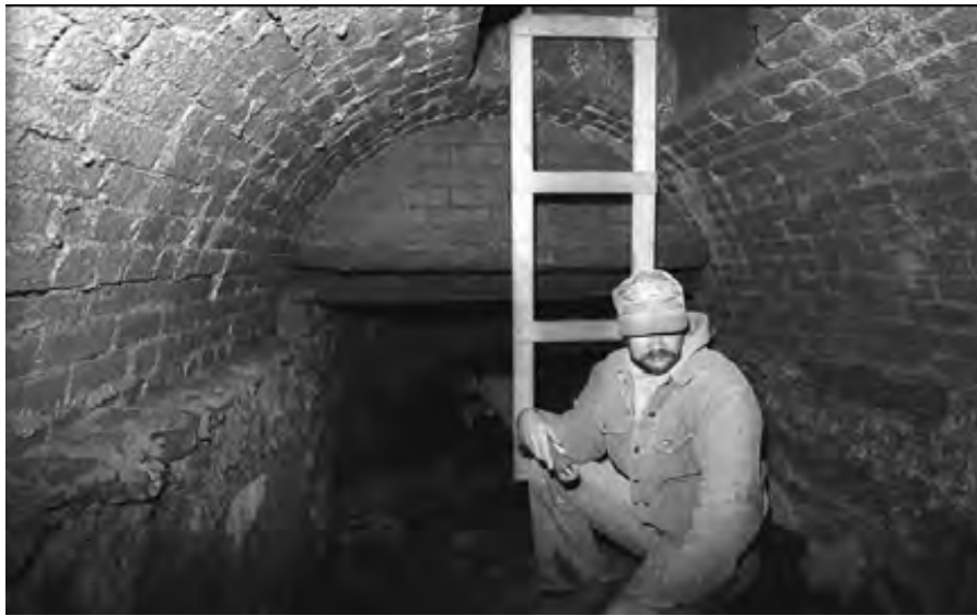
Figure 78. Photograph of the interior of Petty's Run Drain.
