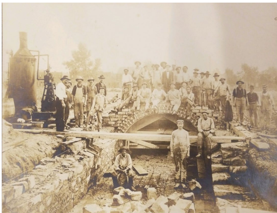
Figure 48. Construction of Newton Creek Line Ditch, with Aaron Ward at center, wearing a bowtie, hat, and suit. Source: Camden County Historical Society, No. 5017.
