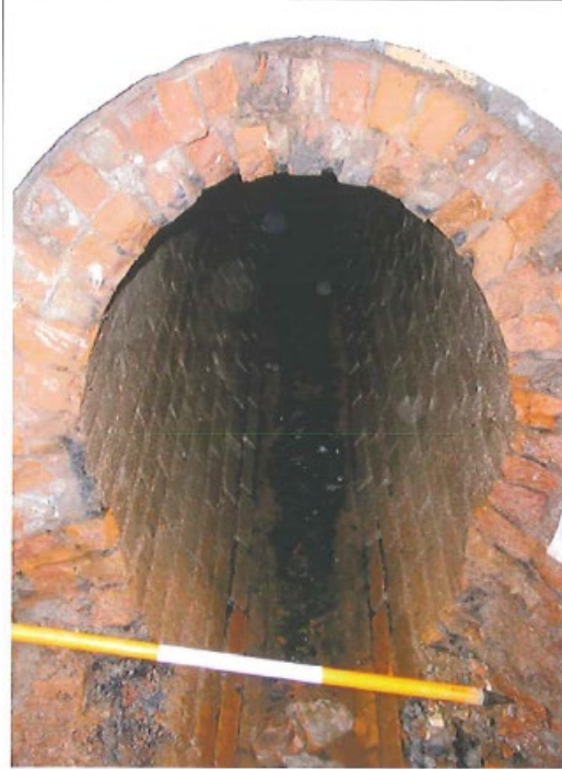
Figure 66. Photograph of the 14th Street egg-shaped sewer.
