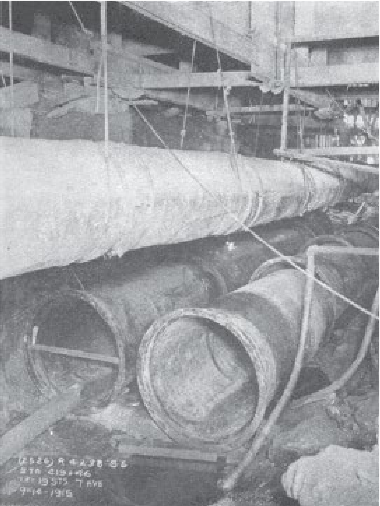
Figure 23. Cast-iron pipes with a 60-inch diameter.
