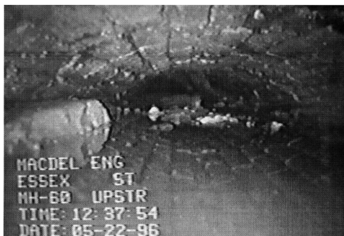
Figure 72. The Essex Street sewer, taken from CCTV footage from 1996.
