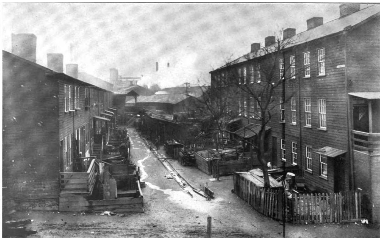
Figure 31. An open drain located between two-family dwellings in Pittsburgh in 1907. Source: F. Elisabeth Croswell, "Painter's Row, The Company House," in The Pittsburgh District, Civic Frontage , ed. Paul Underwood Kellogg (New York: Survey Associates, Inc., 1914). https://www.russellsage.org/sites/all/files/Kellogg_The%20Pittsburgh%20District_o.pdf
