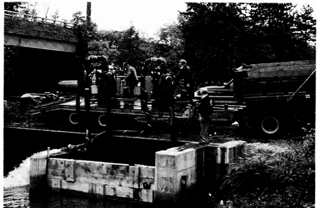
Dewatering operations at the US Route 1 conduit in Trenton.
