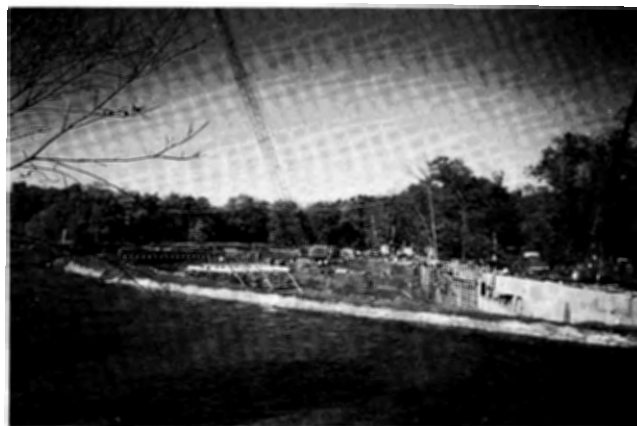
Construction of the "Island Farm" weir downstream of the confluence of the Raritan and Millstone Rivers in Somerset County.
