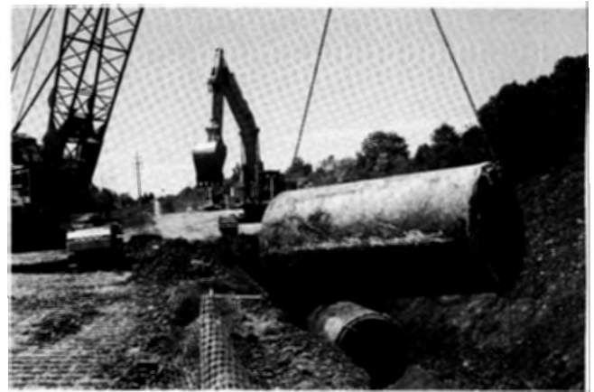
Sections of the 3.6 mile long Round Valley Release Pipeline were replaced.
