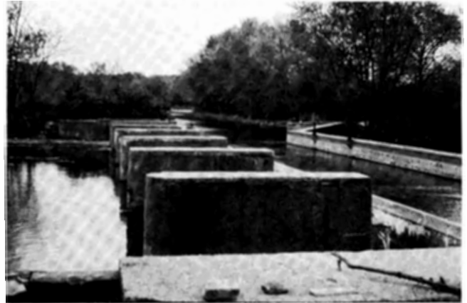
The Carnegie Lake Aqueduct near Princeton, Mercer County.
