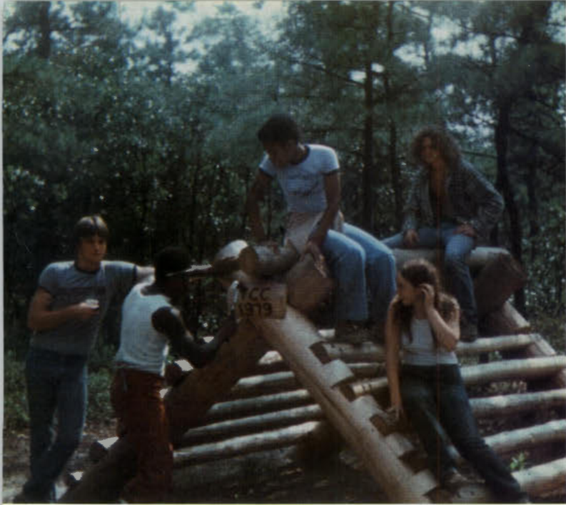
Completion of playground climbing equipment at Rockingham Picnic Area.
