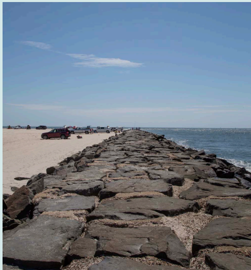
A rocky shoreline located in Brigantine, New Jersey. Rocks can help to reduce sand erosion and protect against storm surge in coastal areas.
