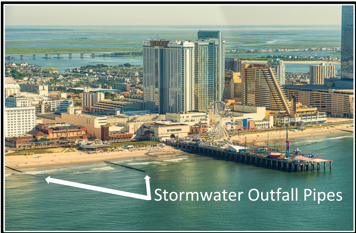
Figure 9: Ocean Stormwater Outfall Pipe, Atlantic City, NJ (Richard Opiekun, NJ Department of Health)
