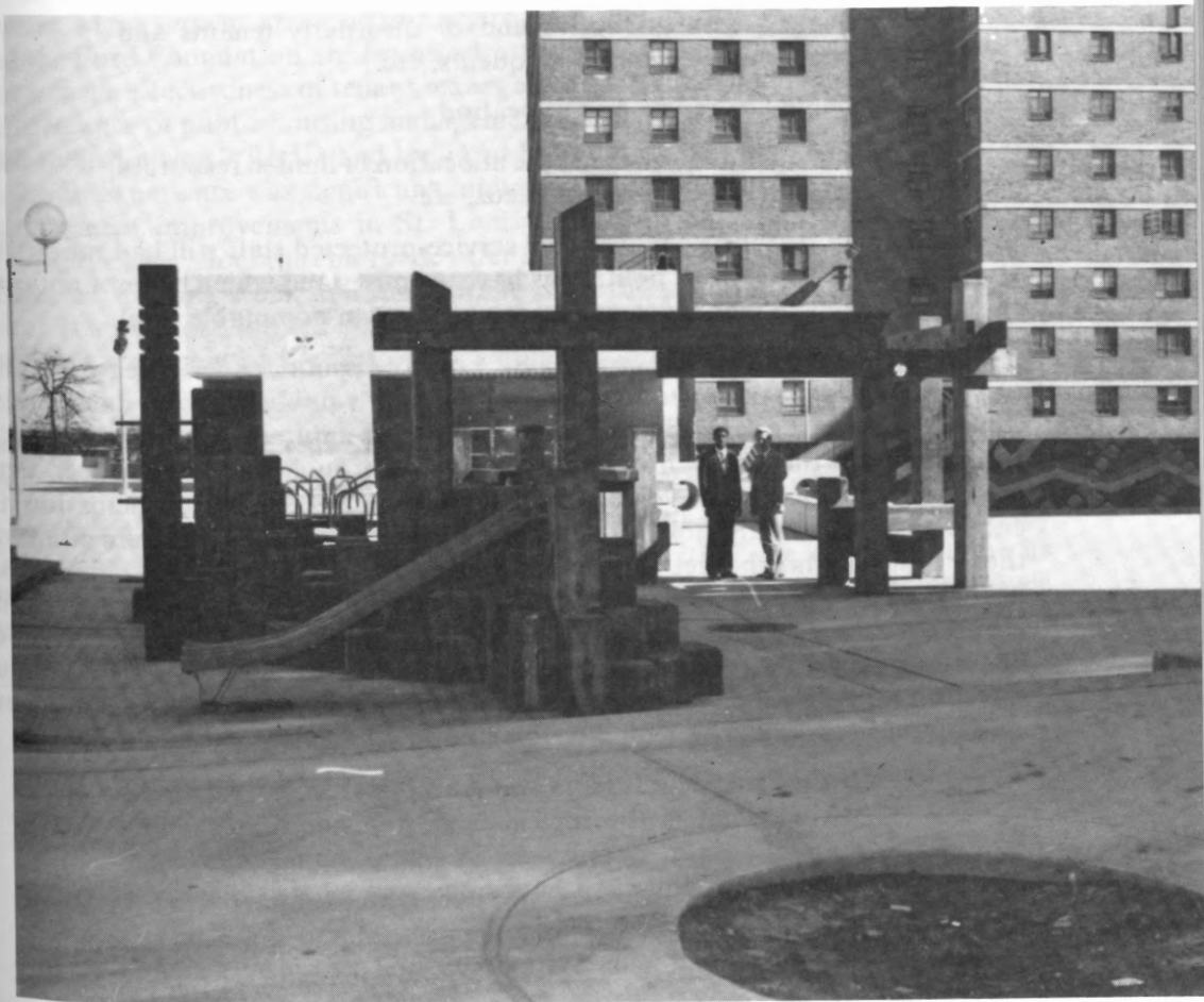
With building security somewhat under control, A. Harry Moore's organization focused their attention on capital planning, in particular the renovation of exterior grounds. (Admiring recently installed recreation equipment, Rev. Robert Blount, Chairman, AHM-TMC Board, left, and Peter M. DePascale, HA Director of Engineering and Construction, 1978.)
