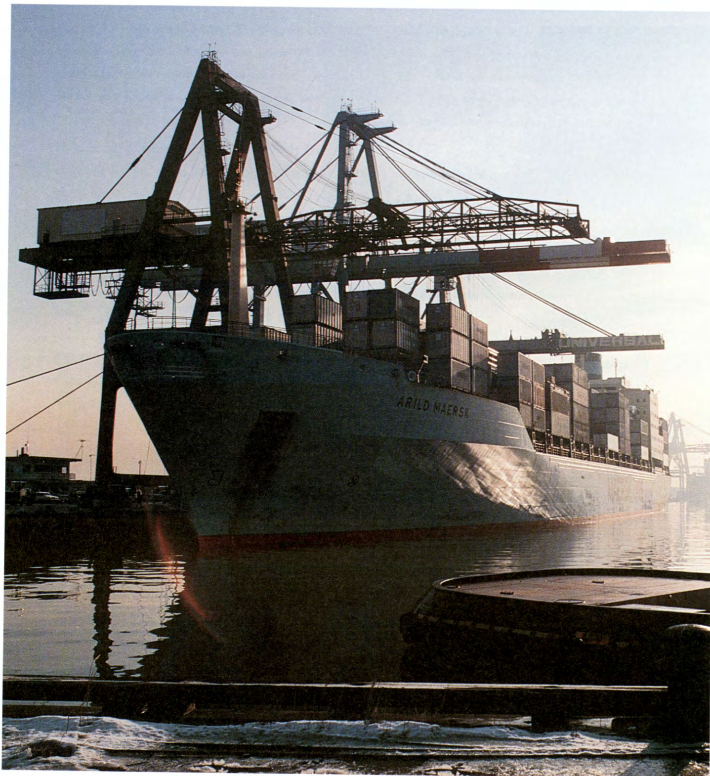
Containership arrives at the Port Newark-Elizabeth Marine Terminal where capital improvements completed in 1991 helped meet the operational needs of tenants.
