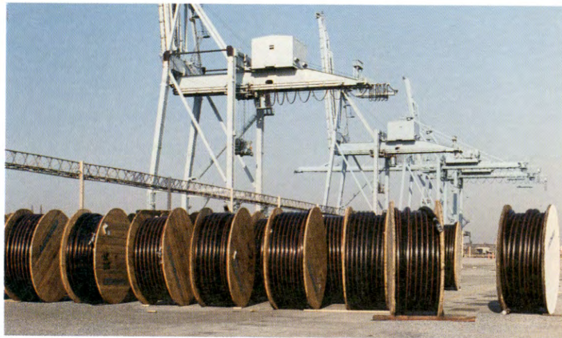
Coils of flexible ducts await installation as part of the renewal of the Howland Hook Marine Terminal's electrical distribution system.
