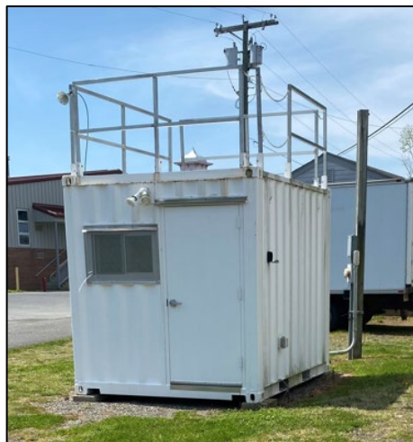
Figure 2-1 Clarksboro Air Monitoring Station
