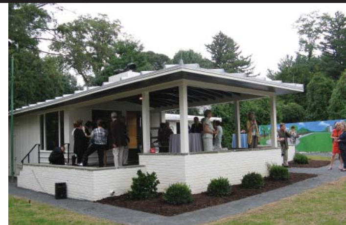
The restored pool house at Historic Morven reopened in September, a project funded by the NJ Cultural Trust.
