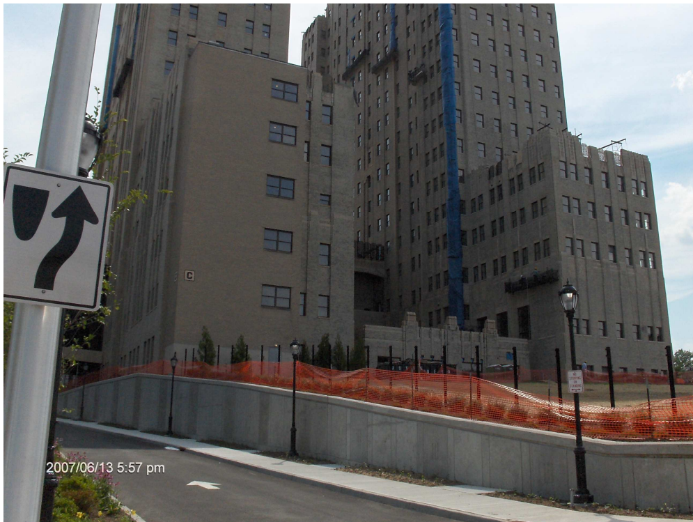
The Beacon condominium development broke ground in March 2006. The conversion of the former Jersey City Medical Center will result in over 300 new condominiums. Photo by Drake Rizzo and Charles Pierson, Jr.
