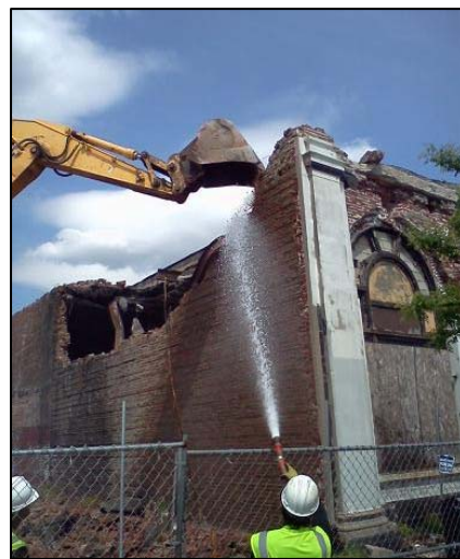
Demolition activities in Jersey City.
