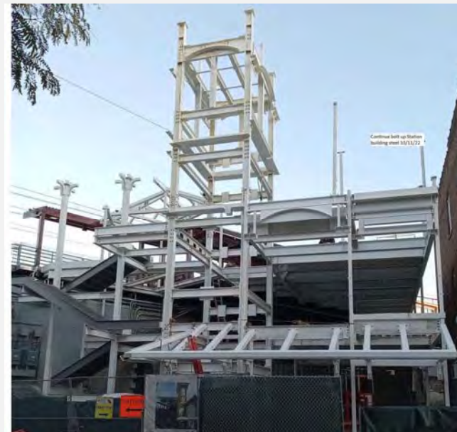
Inbound Station Building Under Construction
